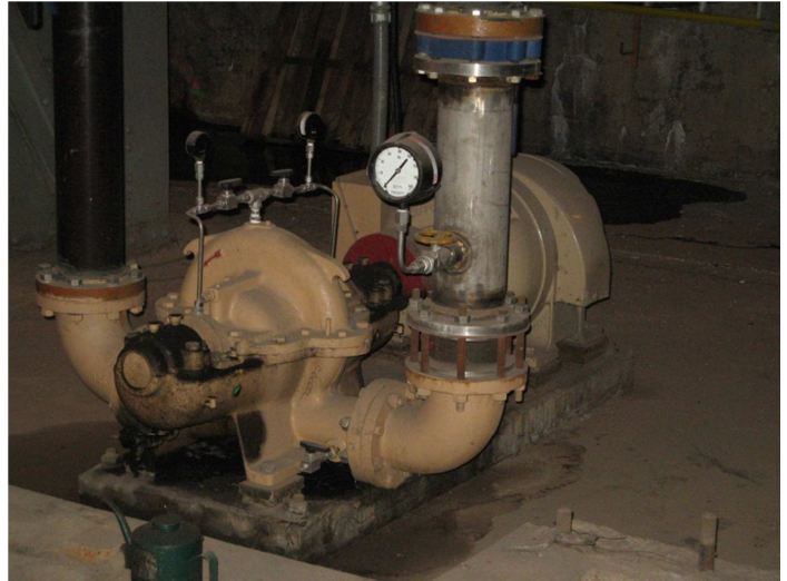
Condensate Transfer Pump
