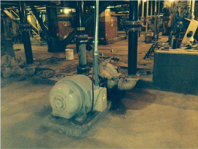
Condensate Transfer Pump
