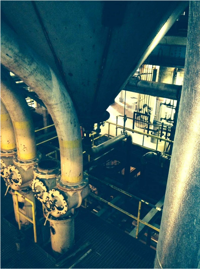
Unit 2 – Coal silo and coal pipes to burners
