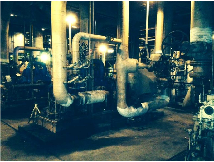
Unit 1A – Boiler Feed Pumps and Turbines
