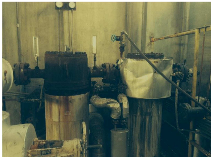
Unit 1B – Feed Water Heaters
