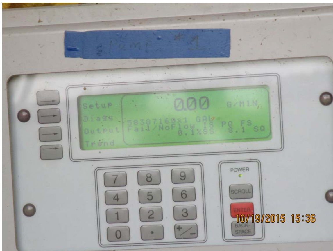
Photo 11 Display screen on properly function Pump No. 1 (left pump on photo 10) 10/19/2015
