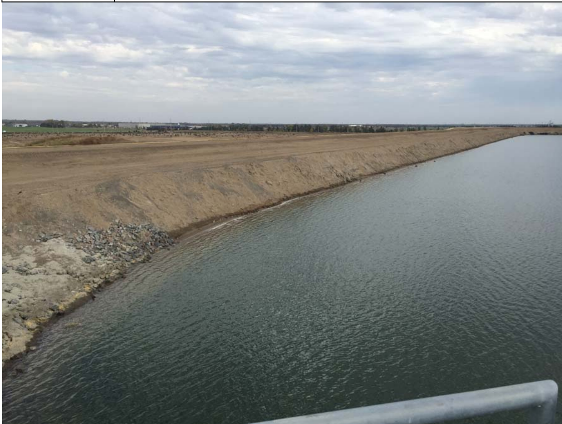
Photo 34 North interior embankment of pond (taken from discharge structure), looking northeast. Freeboard at time of photo: 10.1 feet to top of clay liner, 14.1 feet to top of embankment
