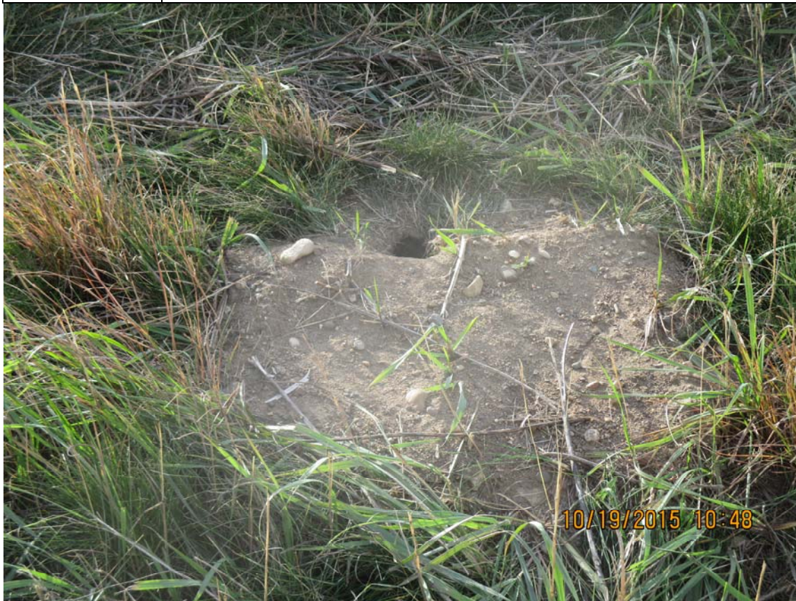
Photo 16 Gopher hole on north embankment
