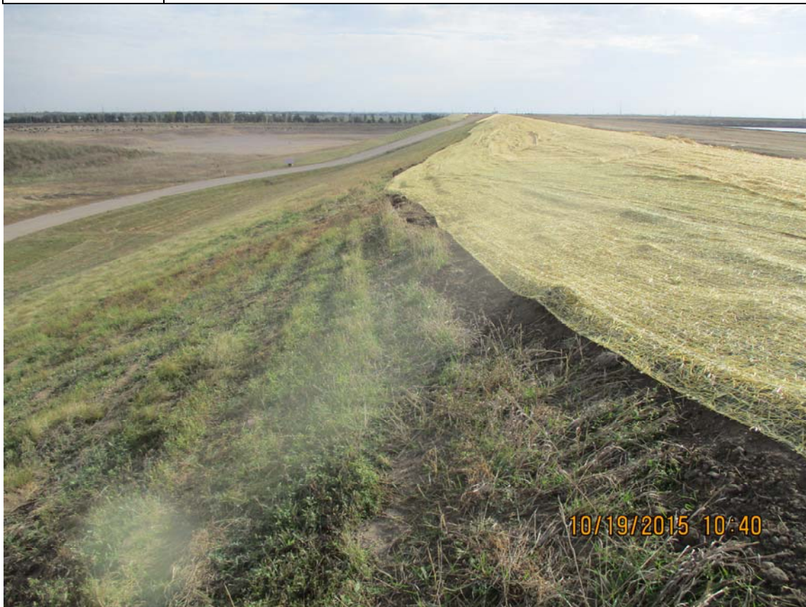
Photo 14 Erosion blanket installed on new pond vertical expansion, looking east
