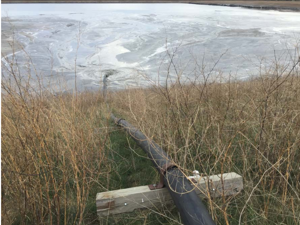
Photo 42 Scrubber pipe (after transition from stainless steel to high density polyethylene) discharging in to south end of pond
