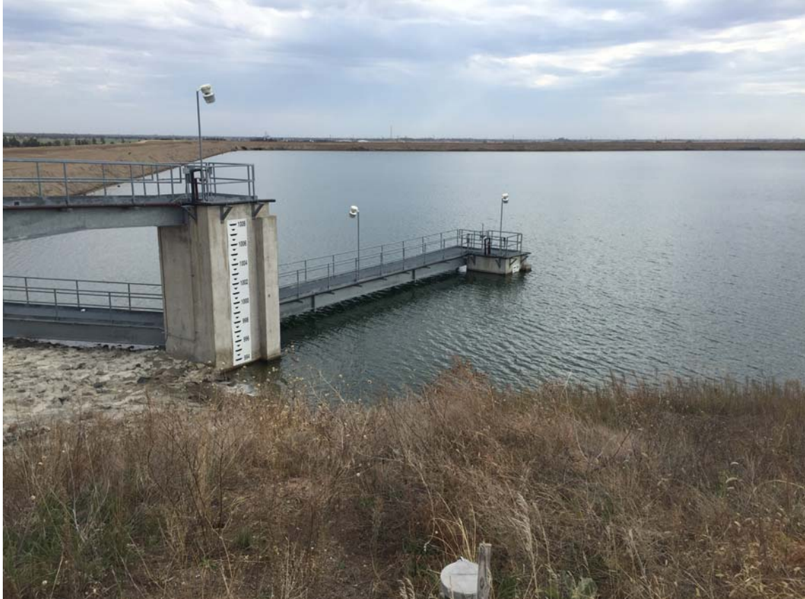
Photo 32 Pond discharge structure in northwest corner of pond. Water level indicates an elevation of 993.2
