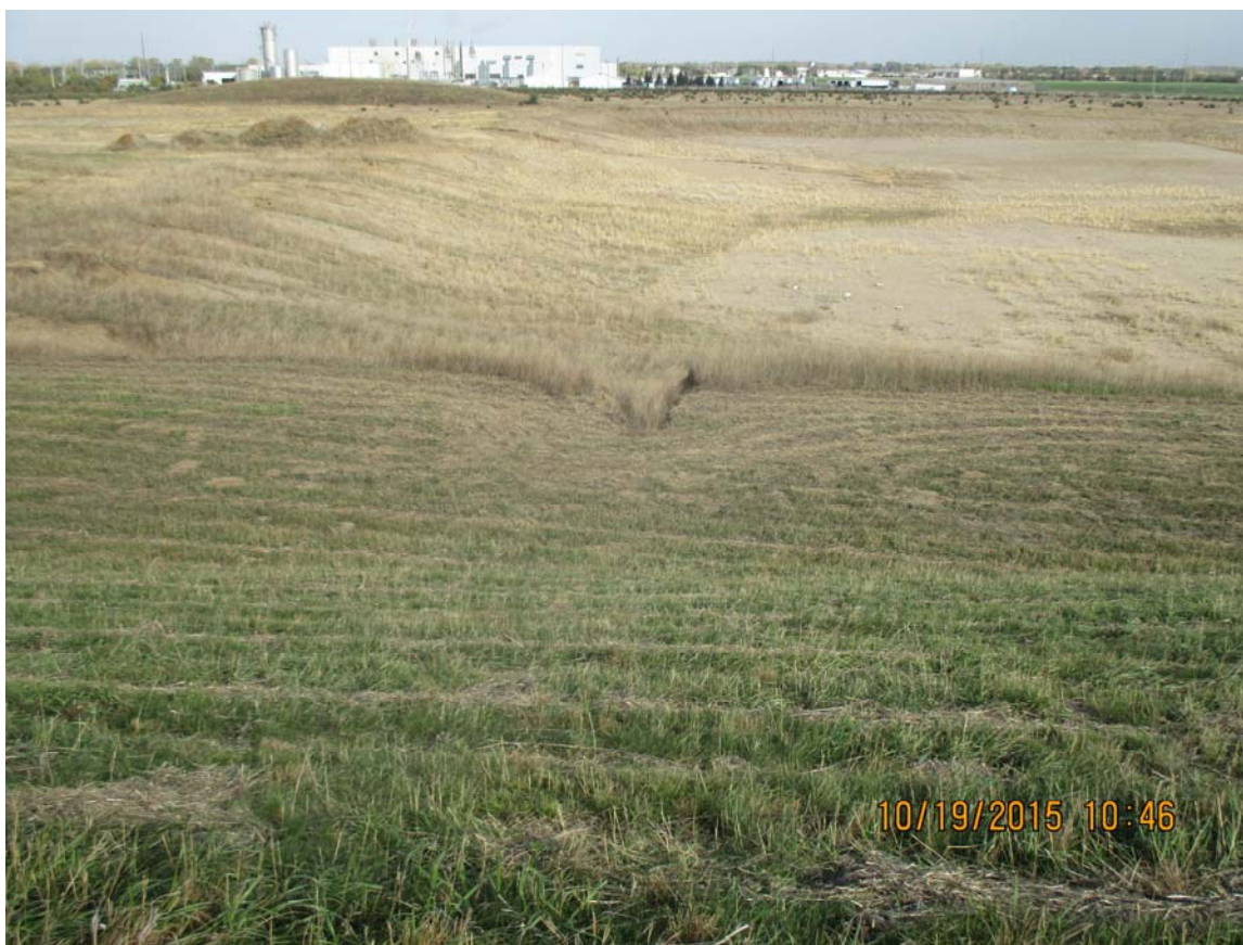
Photo 15 Erosion in the bench between the pond embankment and borrow area.
