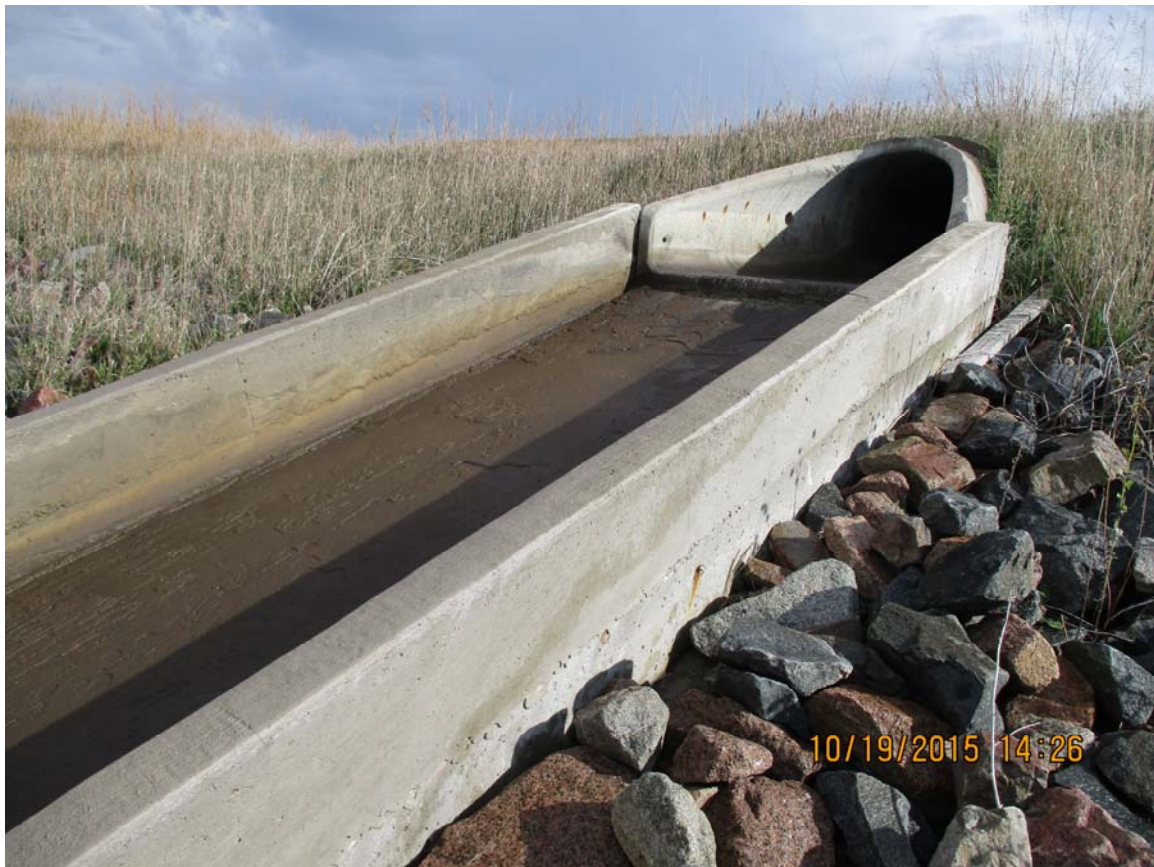
Photo 7 Bottom Ash Pond secondary outlet to Recycle Basin (Primary outlet is below the water level of the Recycle Basin).
