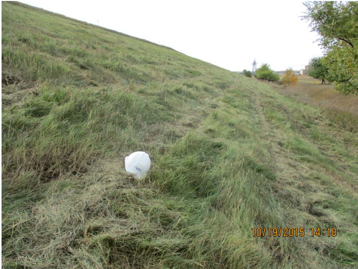
Photo 3 Northern slope, looking west. Hard hat used to shown length of grass (approximately 6 inches).
