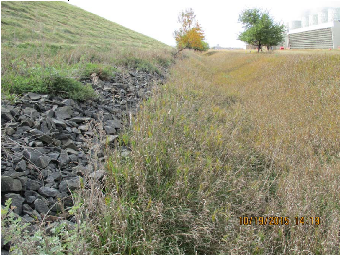
Photo 4 Left: Rirap outlet of embankment toe drain. Right, perimeter ditch, looking west.
