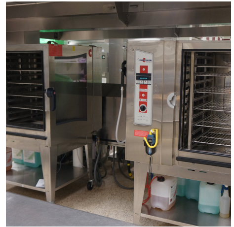
Top: Hot fold holding cabinet Bottom: Combi ovens
