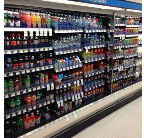
The former open refrigeration cases were inefficient.
