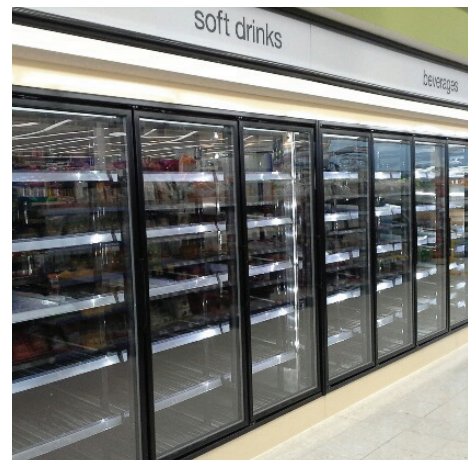
"Close the case" initiative added doors to refrigerated section to improve efficiency.
