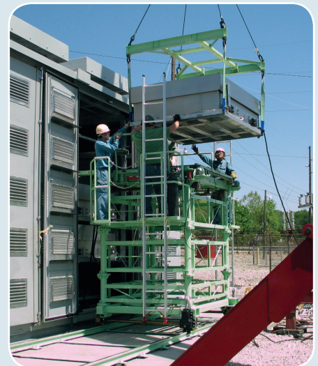
Lifting a battery module into place Photo courtesy of S&C Electric Company
