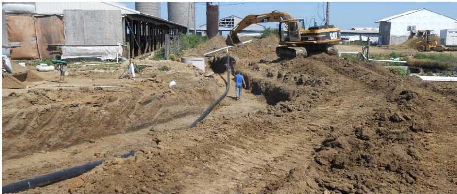
Photo 4: Laying in the pipe that brings the manure to the digester
