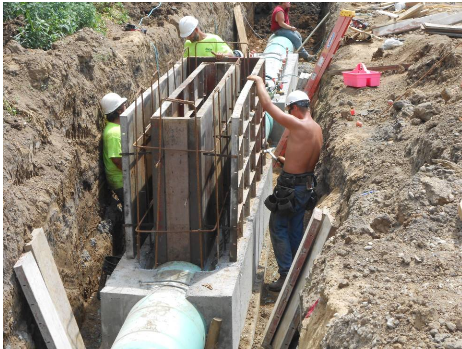
Photo 2: Workers preparing one of the manure drops
