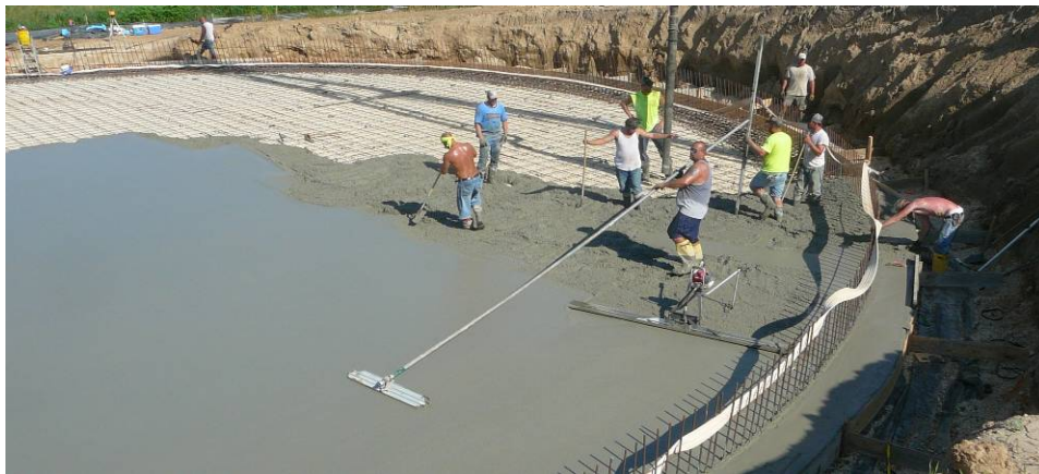
Photo 5: Pouring the floor of the digester
