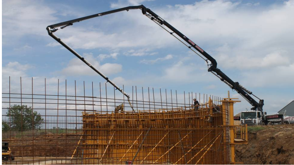
Photo 6: Construction of the digester walls
