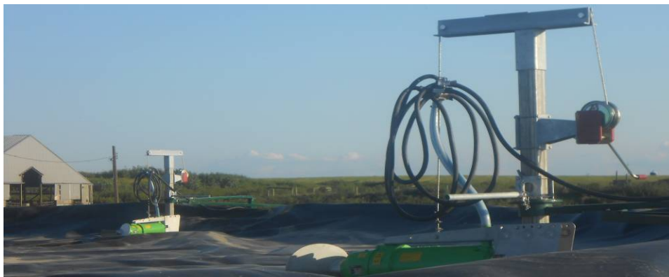
Photo 8: Agitators to stir the manure in the digesters
