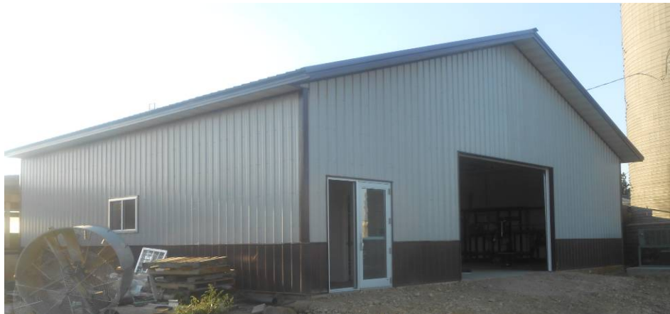
Photo 12: The building that houses the electrical generation equipment
