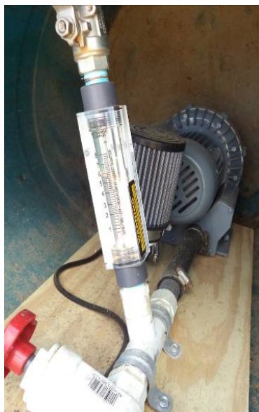
Photo 4: A very simple, but very precise, introduction of a measured amount of oxygen into the digester vessel converts the H_2S from a gas to a granule.
