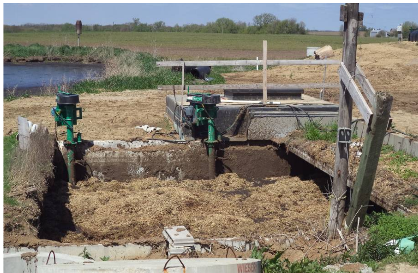
Photo 6: The manure flows by gravity from all of the collection gutters into the central collection pit.
