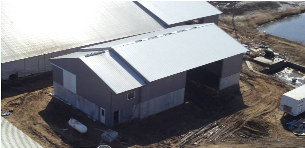
Photo 9: Digested slurry is processed through a screw press separator located in the separator building. Solids are also collected and stored in this building.
