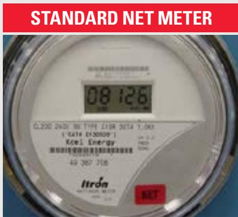
This net meter rolls backwards when your PV system is generating more electricity than you are using in your home and it rolls forwards when you are pulling electricity into your home from the grid. During a 24 hour time frame this meter has the potential for back and forth motion. At the end of the billing cycle we use the meter reading to send you a net summary of your electric consumption or production.
