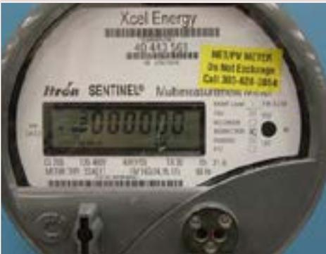
This meter separately measures the energy being pulled into your home from the grid and the energy your system is pushing out onto the grid.
