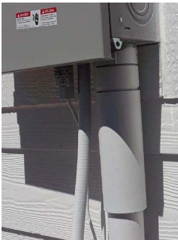
Figure 1: Expansion Joint Installation
