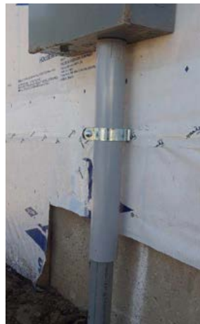
Figure 2: Expansion Joint Installation
