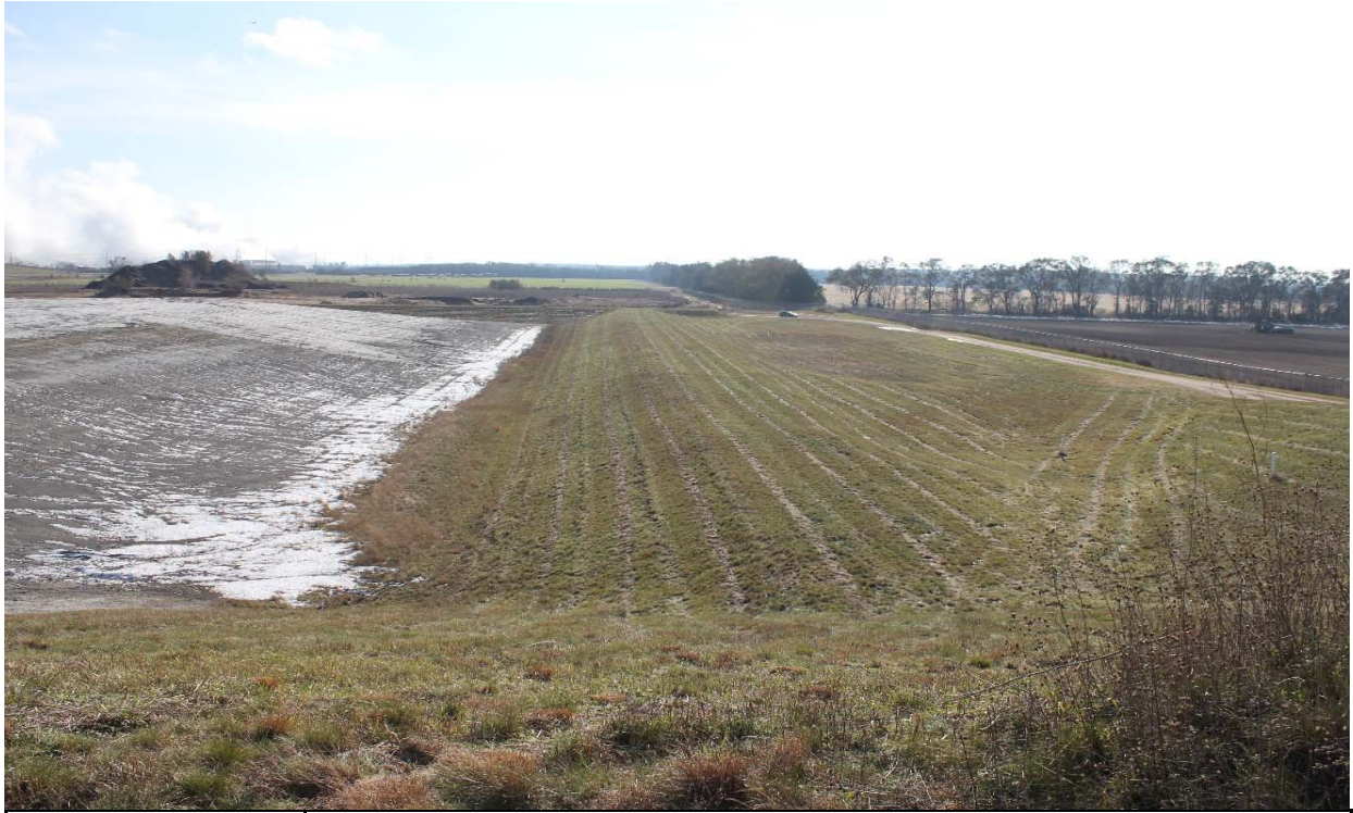
Photo 7 Run-on/run-off containment berm along west side of landfill, looking south. 11/8/2017
