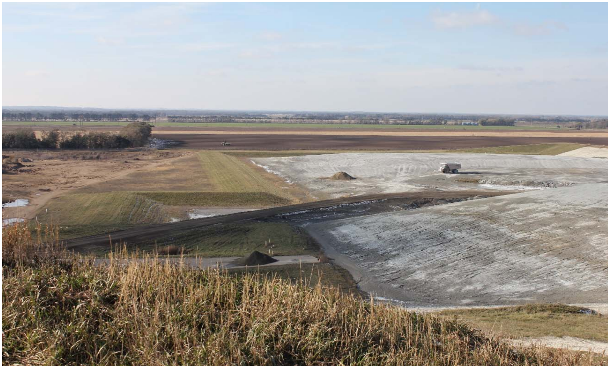
Photo 4 Run-on/run-off containment berm along south side of open area, looking west. 11/8/2017
