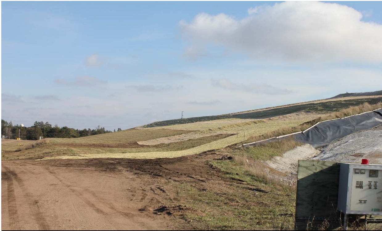
Photo 11 Newly installed final cover along the north side of the landfill, looking east. 11/8/2017
