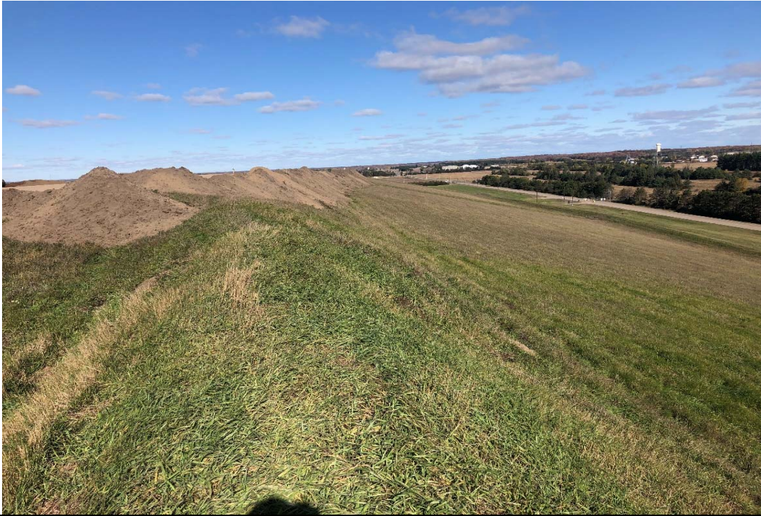
Photo 1 Left: construction of new final cover. Right: existing final cover 10/24/2019 (constructed in 2017), looking north.
