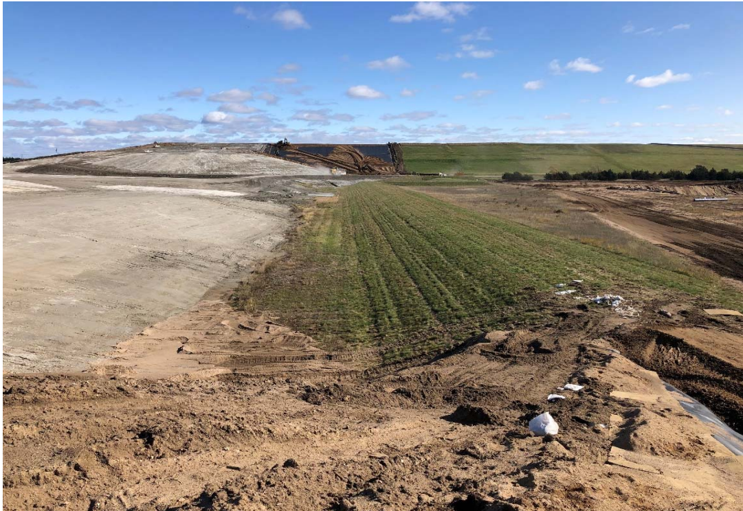
Photo 2 Run-on/run-off control berm, looking east. 10/24/2019
