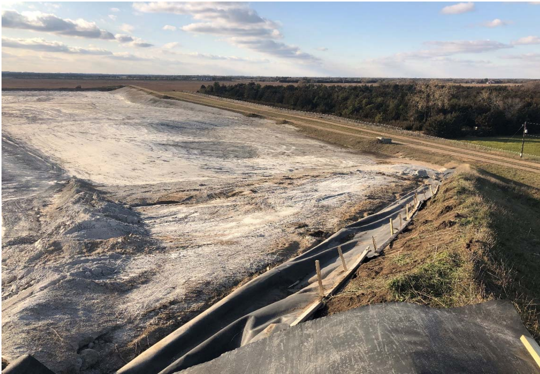
Photo 7 Run-on/run-off containment berm along east side of landfill, looking west. 10/24/2019
