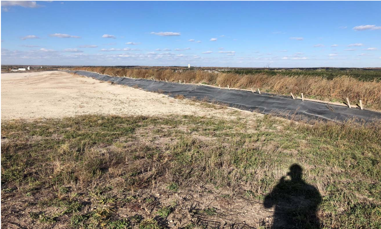
Photo 3 Leachate run-off containment flap along edge of final cover, looking northeast. 10/22/2018
