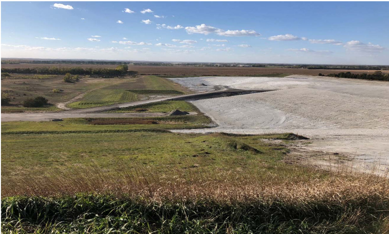
Photo 4 Run-on/run-off containment berm along south side of open area, looking west. 10/22/2018
