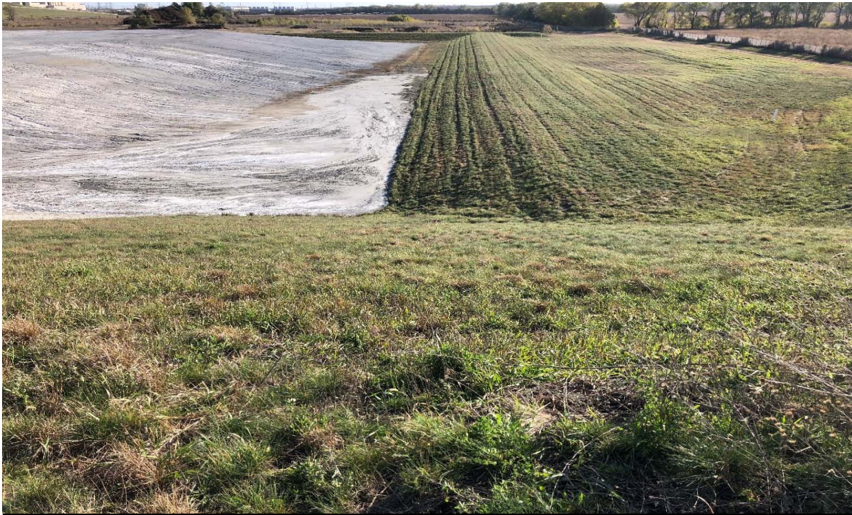
Photo 7 Run-on/run-off containment berm along west side of landfill, looking south. 10/22/2018
