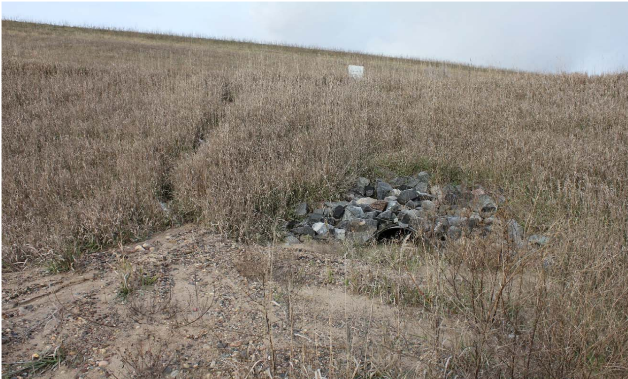
Photo 3 Stormwater outlet and small eroded channel on outer east slope of south embankment, looking northwest. 11/8/2017
