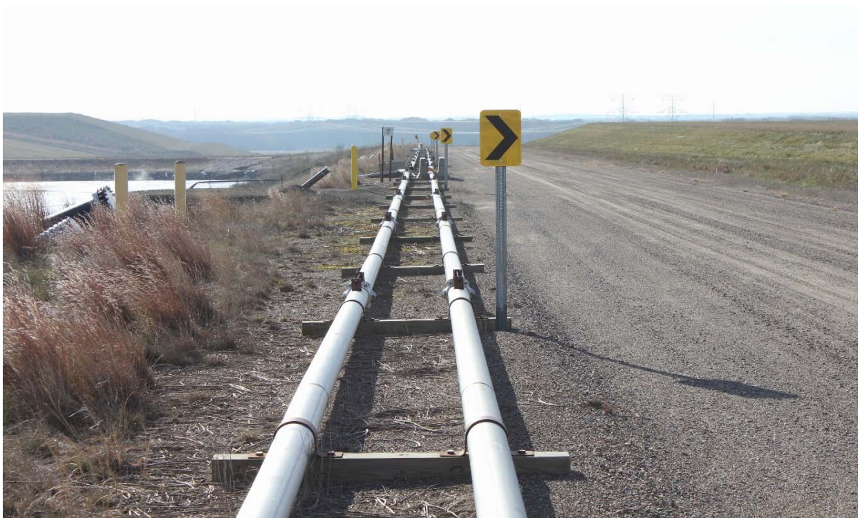
Photo 30 Foreground: Pond stainless steel scrubber solid pipes. Middle-left: CCR angled well. 11/8/2017
