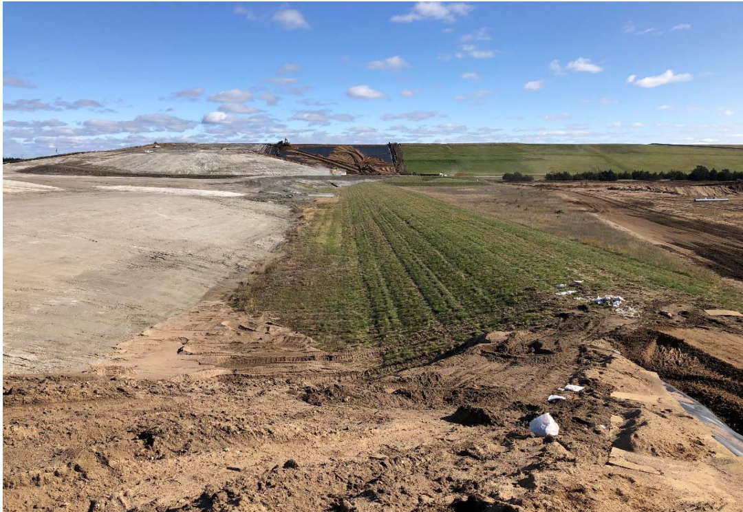
Photo 2 Run-on/run-off control berm, looking east. 10/24/2019
