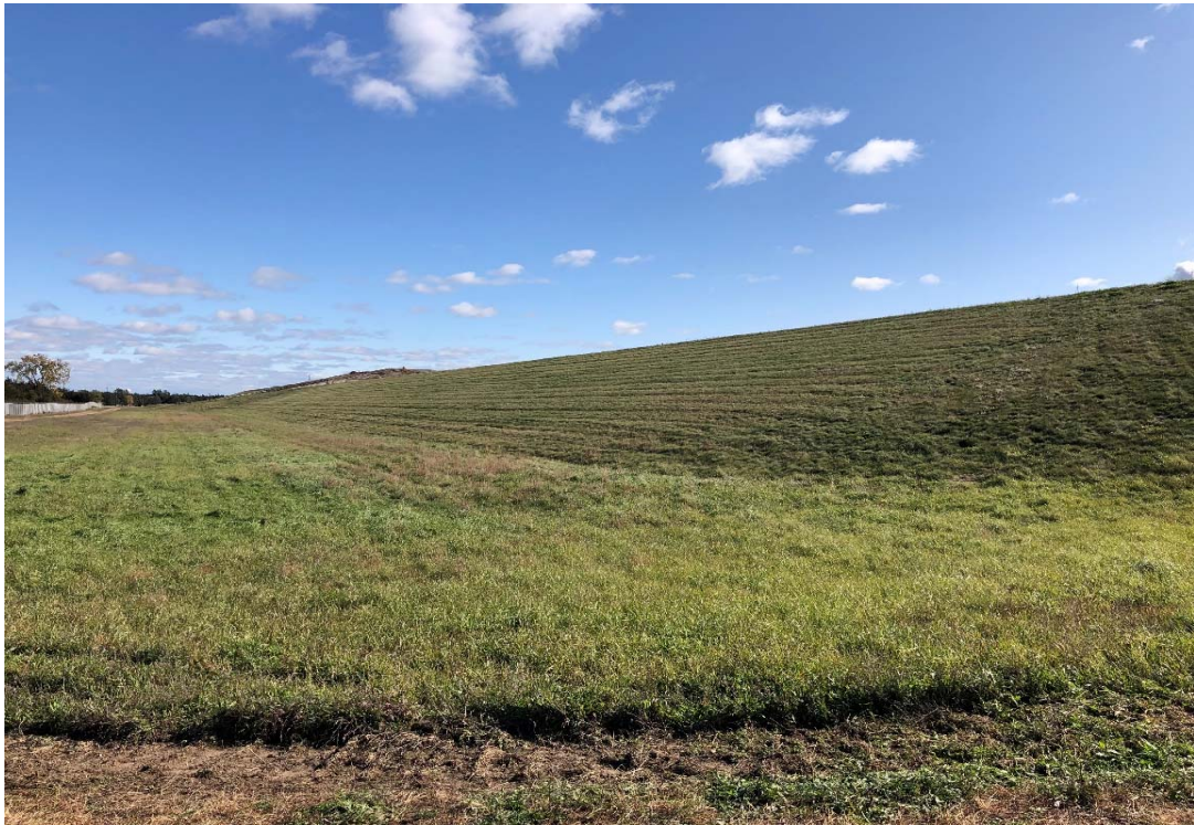
Photo 5 Exterior of north berm, looking east. 10/24/2019
