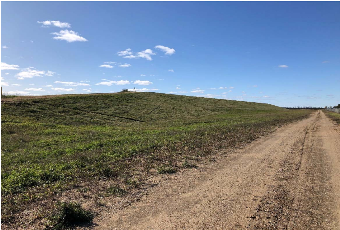
Photo 6 Exterior of north berm, looking west. 10/24/2019
