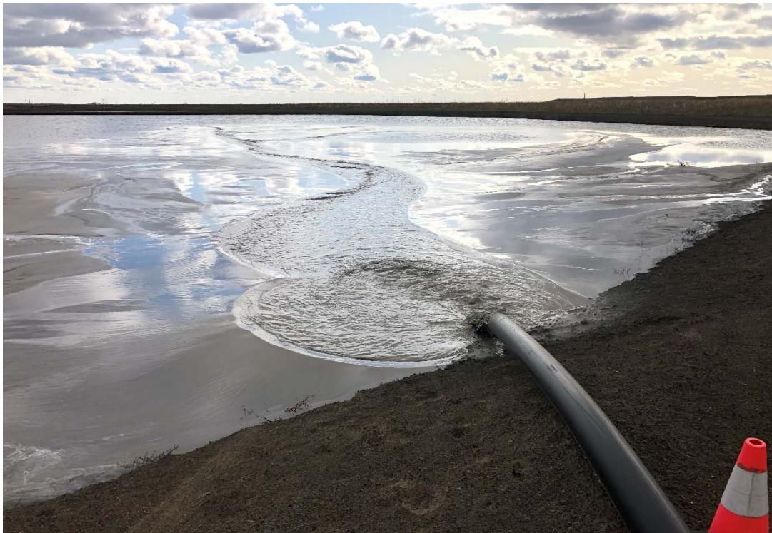
Photo 22 Scrubber solids discharge pipe, looking east. 10/24/2019
