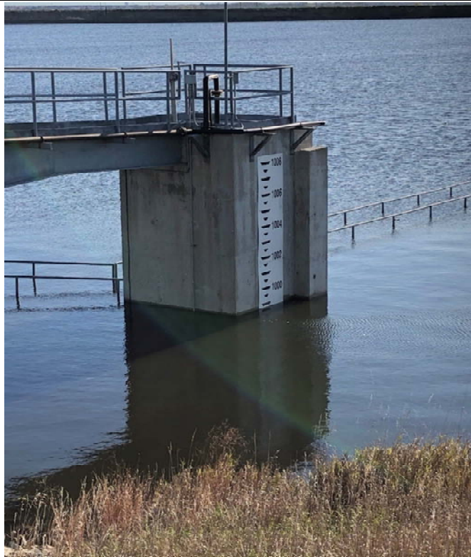
Photo 12 Pond 3 staff gauge, reading an elevation of 998.75 feet (mean sea level). 10/24/2019
