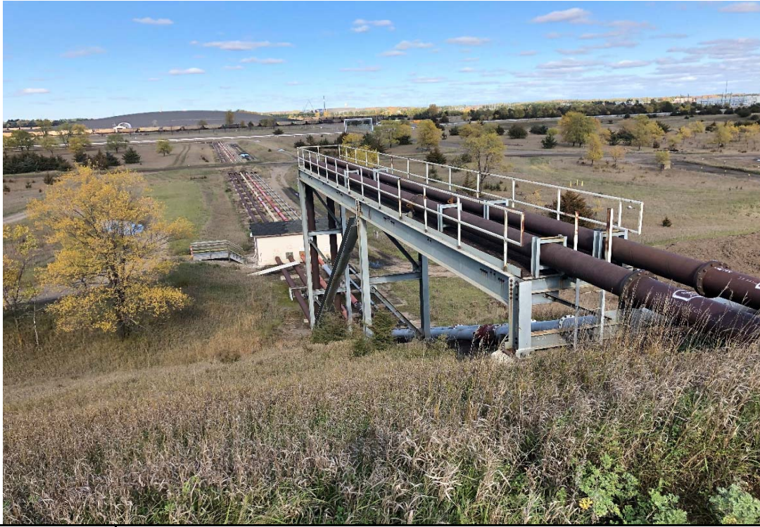
Photo 1 Bottom ash and scrubber pipes, looking northeast. 10/24/2019
