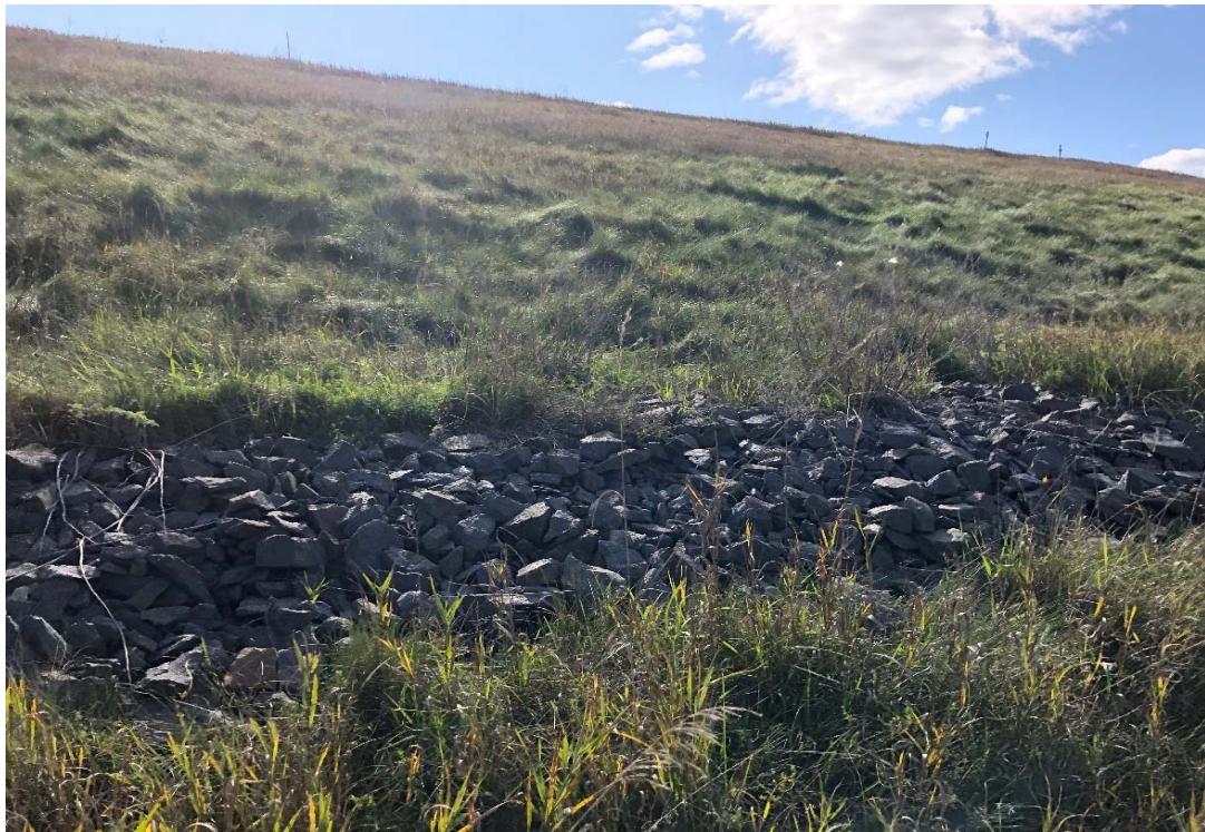
Photo 14 Toe drain of north slope, looking south. 10/24/2019
