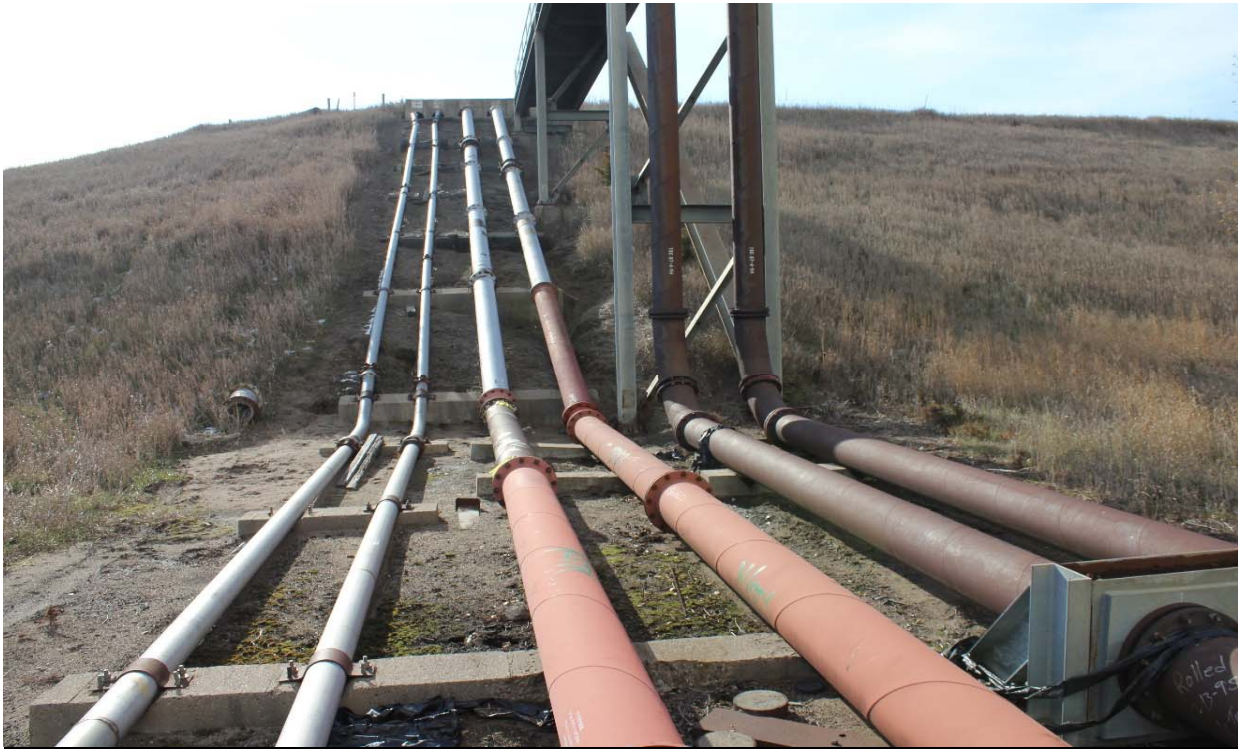
Photo 1 Bottom ash and scrubber pipes, looking south. 11/8/2017
