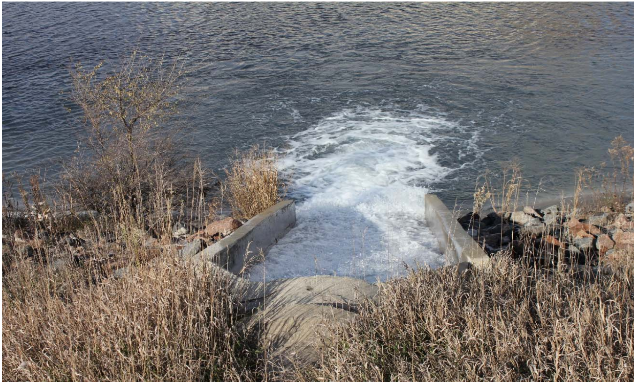
Photo 5 Bottom Ash Pond secondary outlet to Recycle Basin (Primary outlet is below the water level of the Recycle Basin). 11/8/2017
