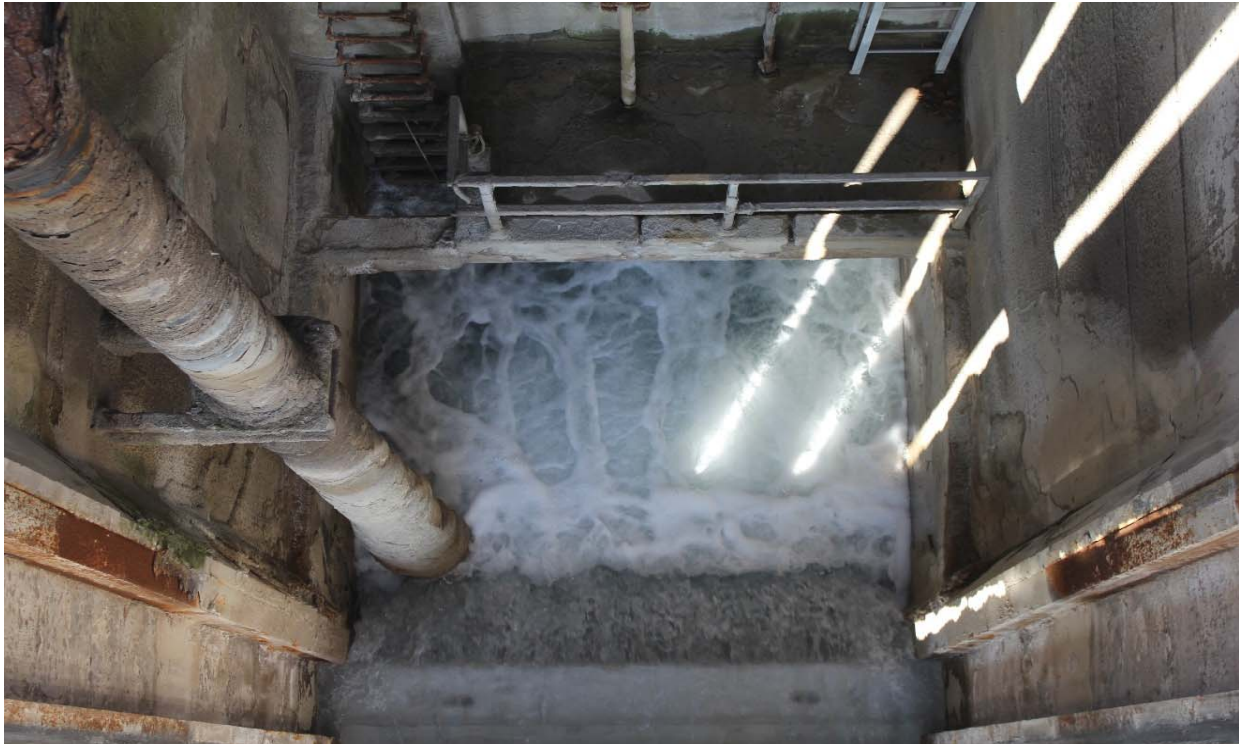
Photo 9 Photo from inside the discharge structure. Shows stop-log metal channels and water flowing over concrete stop-log at the bottom of the channel. 11/8/2017
