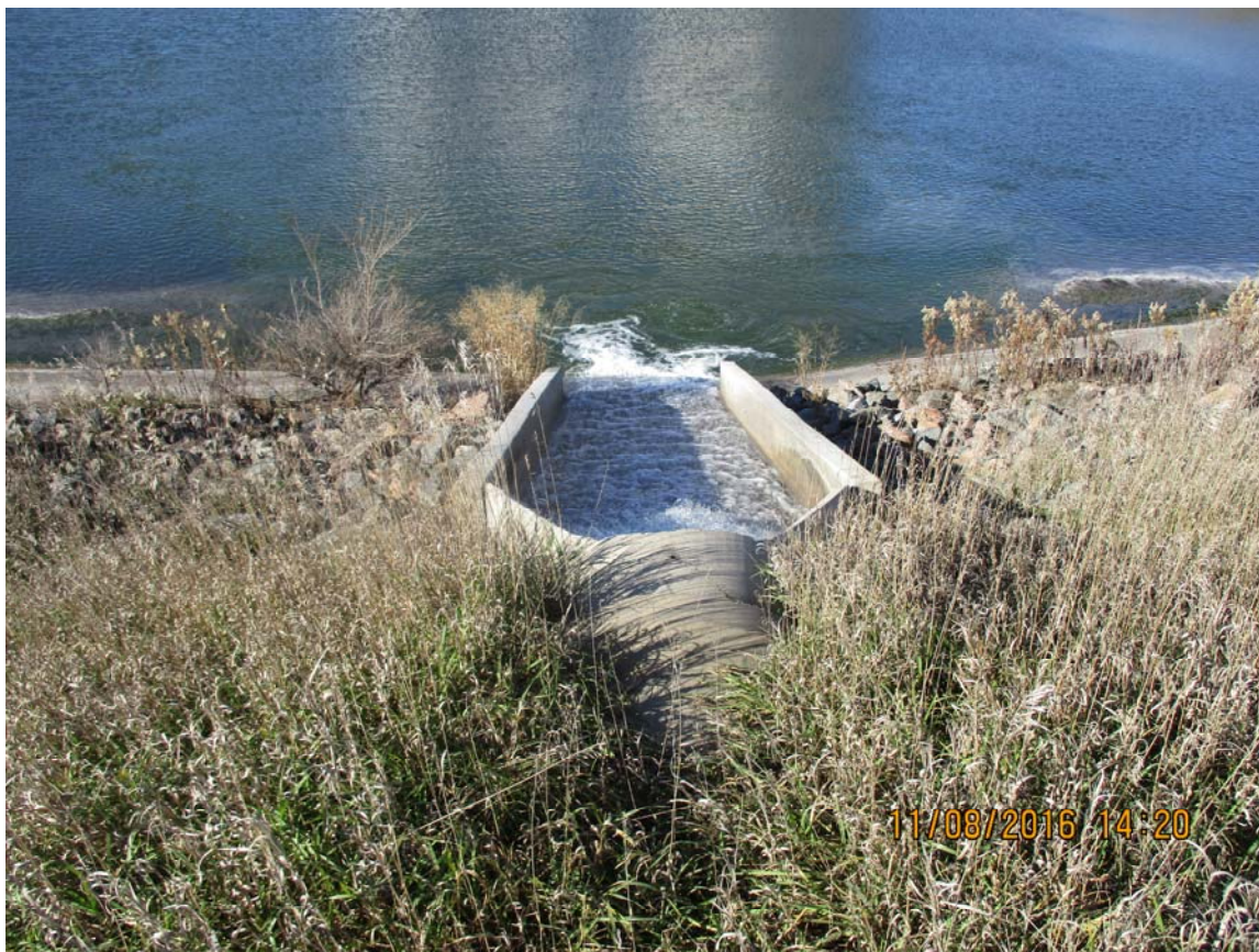
Photo 5 Bottom Ash Pond secondary outlet to Recycle Basin (Primary outlet is below the water level of the Recycle Basin).
