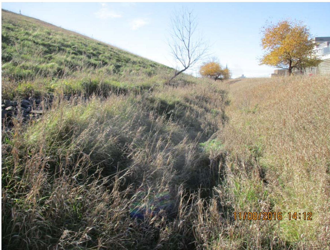
Photo 3 North embankment and riprap toe drain, looking west.
