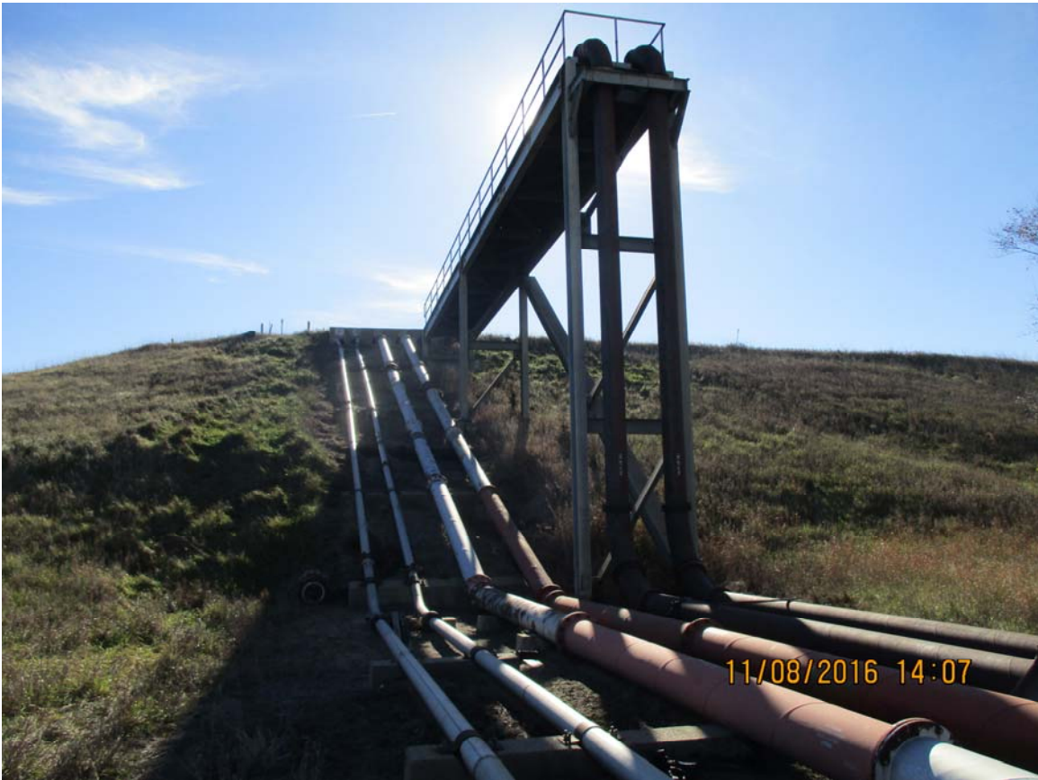
Photo 1 Bottom ash and scrubber pipes, looking south 11/8
