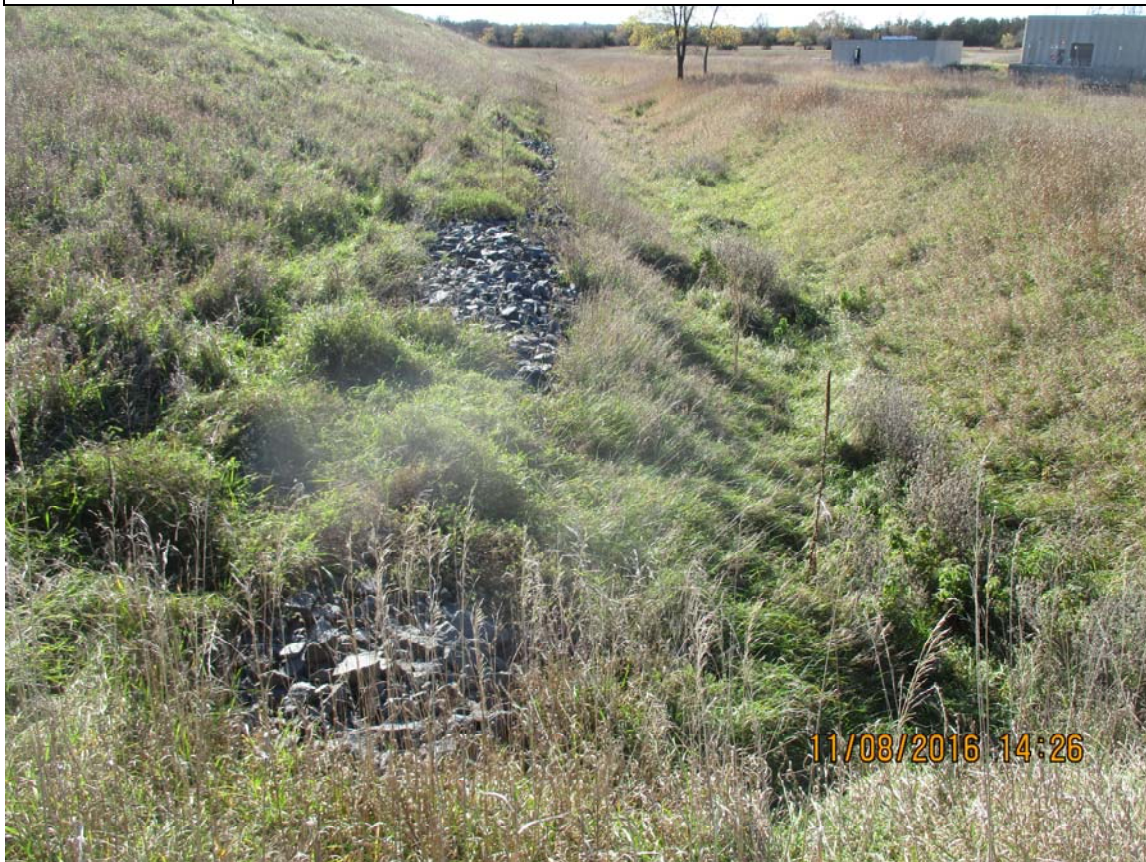
Photo 6 Northwest embankment riprap toe drain, looking southwest.
