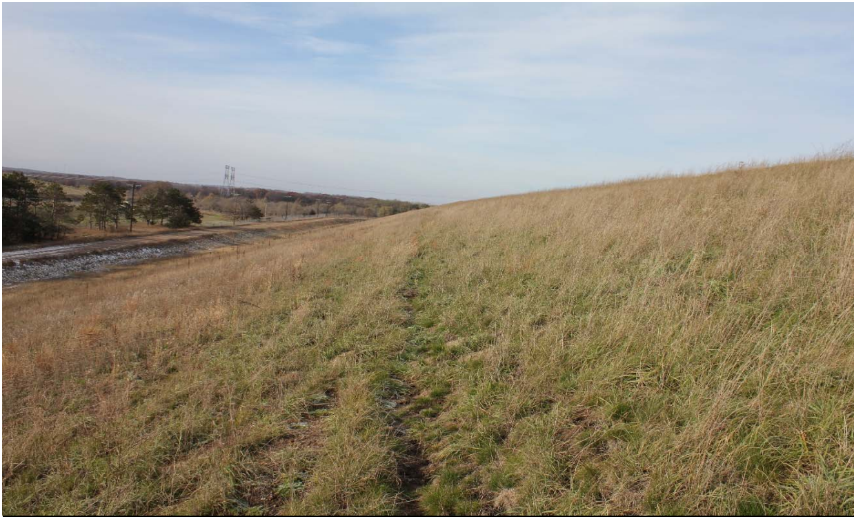
Photo 21 Mid-slope of south embankment, looking west. 11/8/2017
