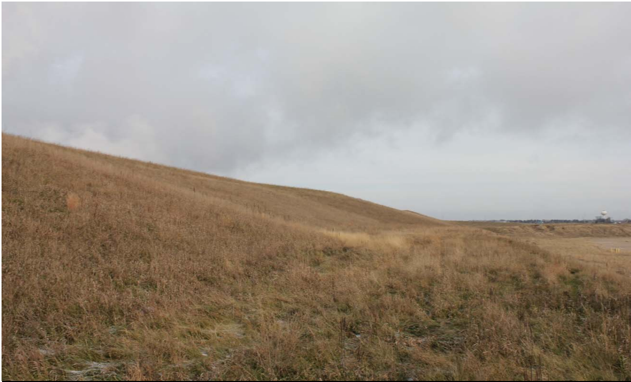
Photo 15 Pond east embankment, looking north. 11/8/2017
