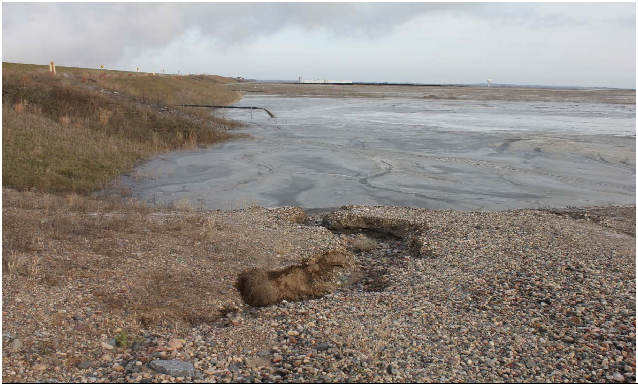
Photo 19 Pond interior west embankment, looking north. 11/8/2017
