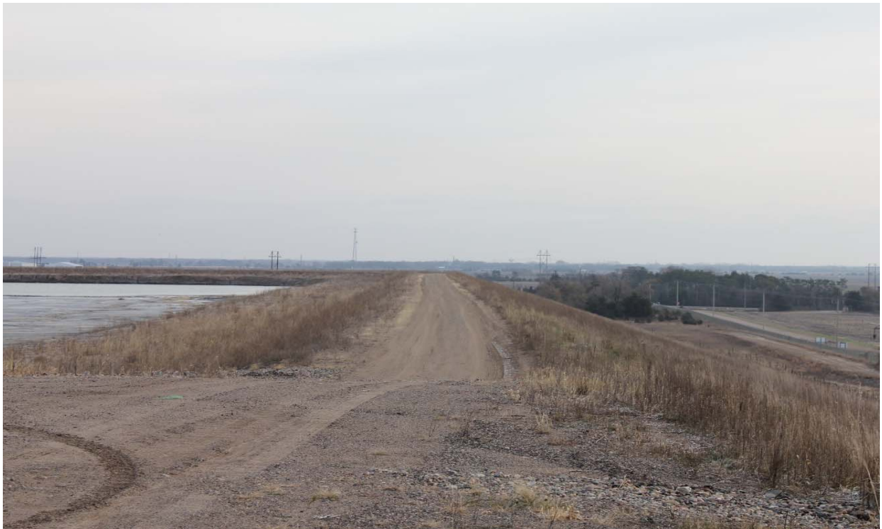
Photo 20 Top of pond south embankment, looking east 11/8/2017
