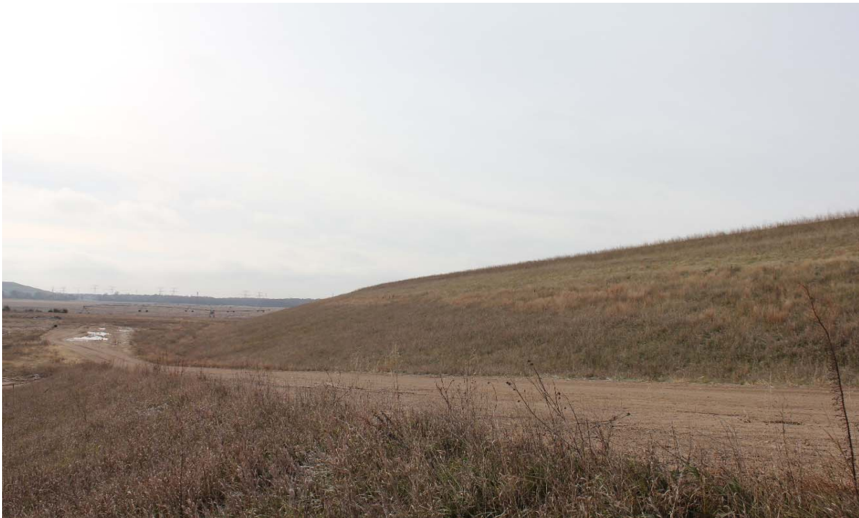
Photo 22 Pond southeast ramp and embankment, looking south. 11/8/2017
