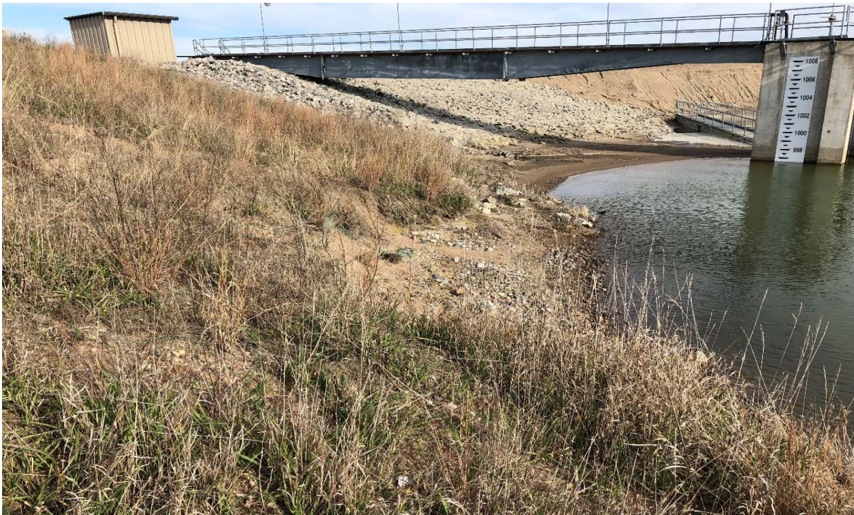
Photo 28 Interior embankment of northwest corner, looking northeast. Pond water level staff gauge (shown at approx. 996.5 feet of elevation mean sea) 10/22/2018
