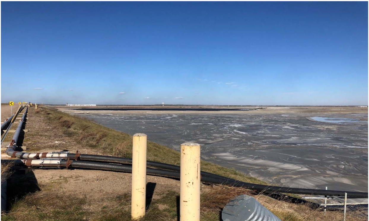
Photo 30 Pond west embankment interior, looking northeast. Left: Pond stainless 10/22/2018 steel scrubber solid pipes. Bottom: dewatering pipe clean-out.
