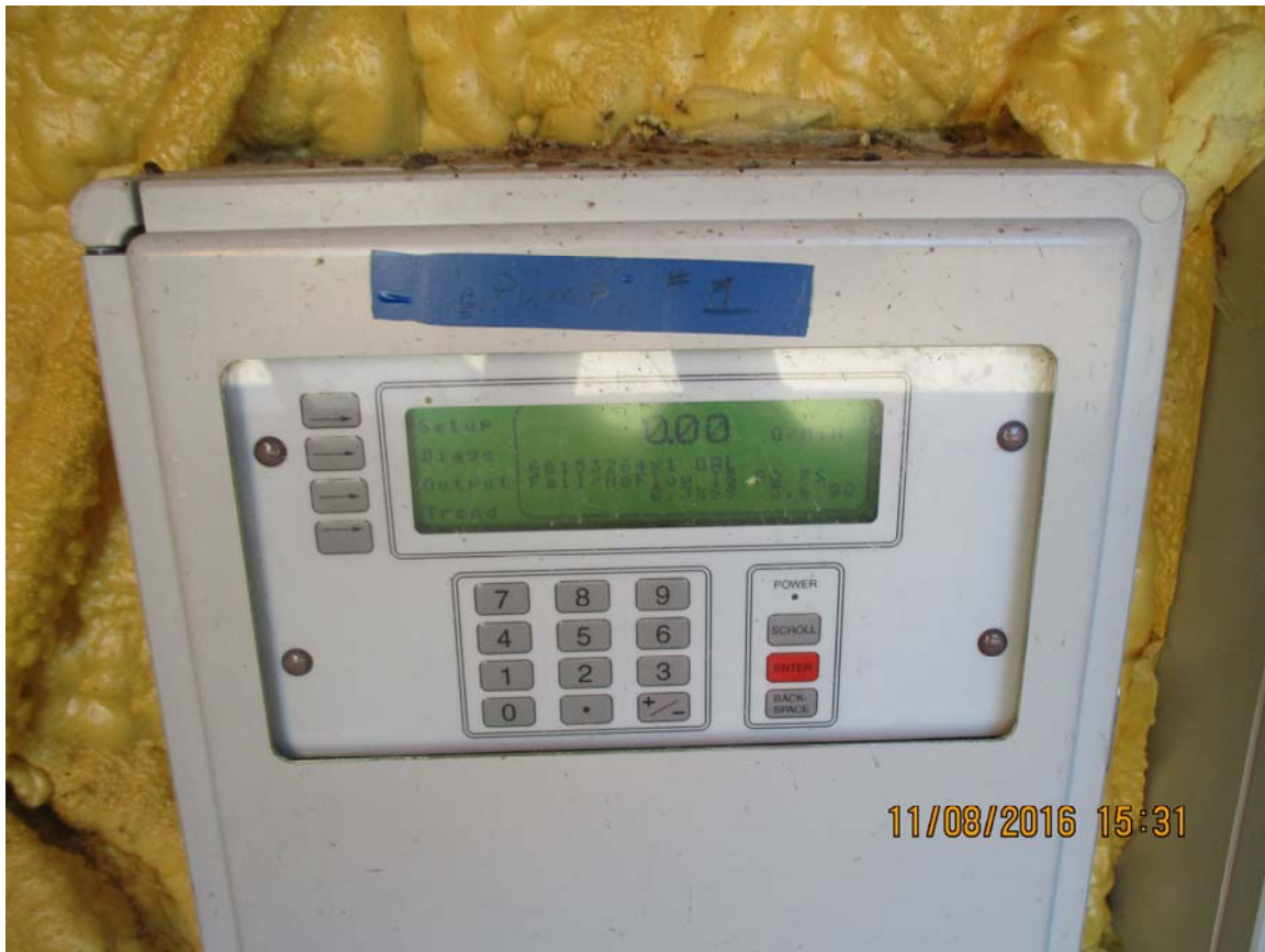
Photo 9 Display screen on properly function Pump No. 1
