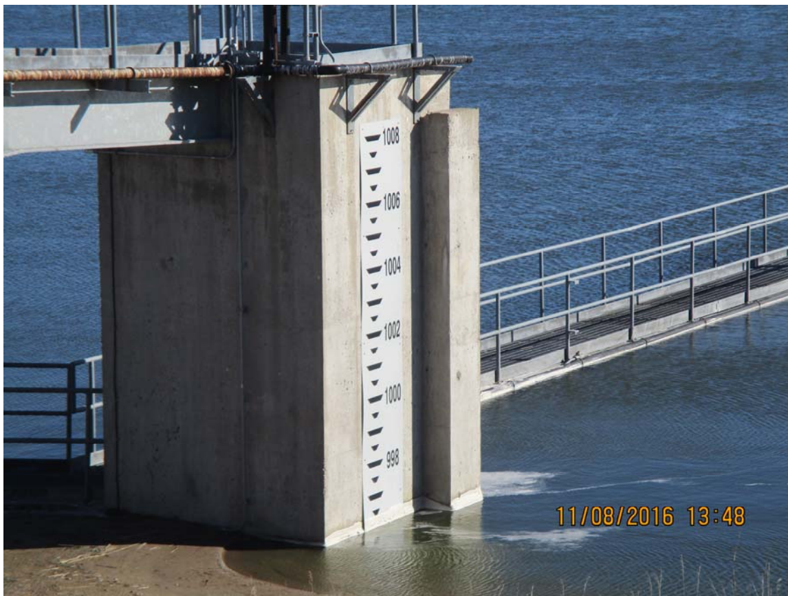
Photo 27 Pond water level staff gauge (shown at approximately 996 feet of elevation mean sea level)
