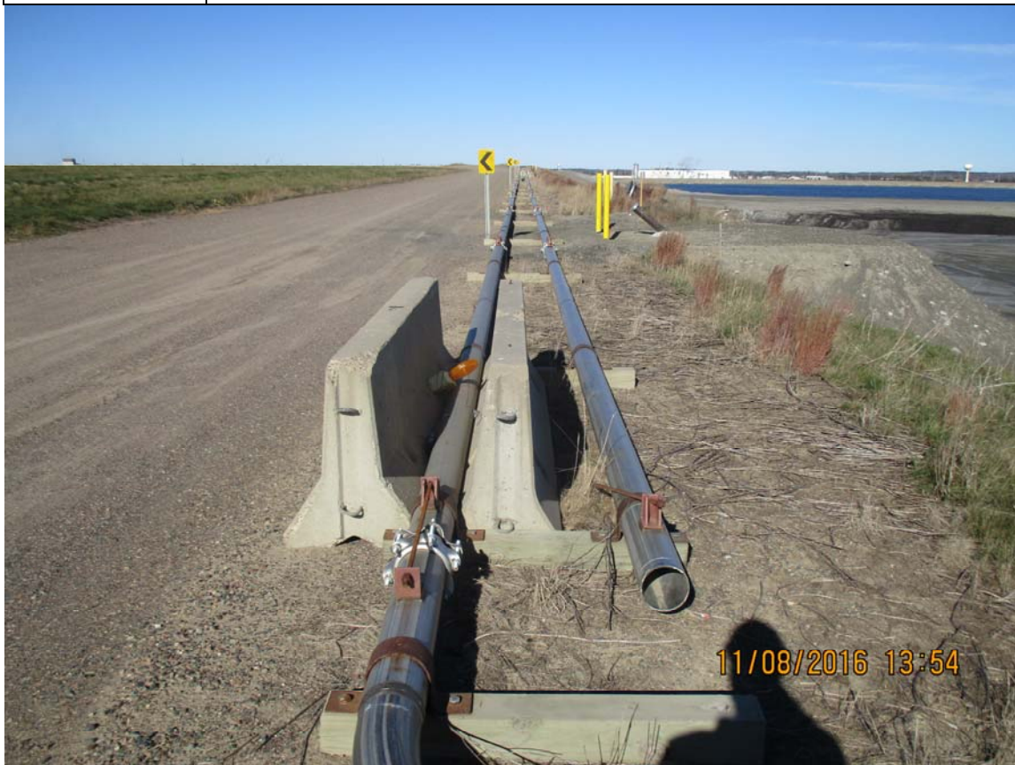
Photo 30 Foreground: Pond stainless steel scrubber solid pipes. Middle-right: newly installed CCR angled well
