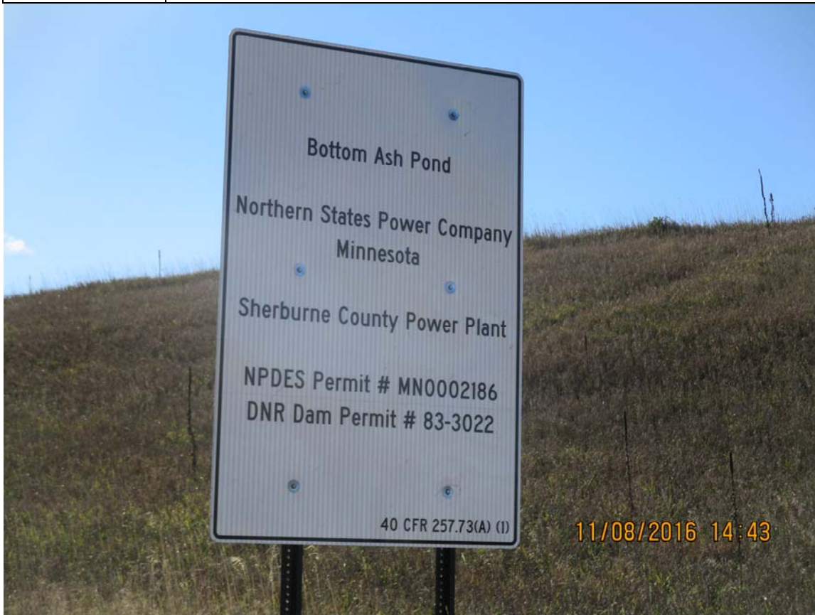
Photo 16 CCR Unit identification marker placed in accordance with Section 257.73
