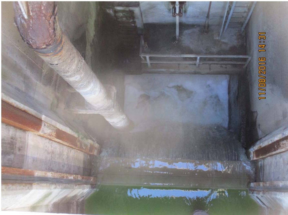
Photo 9 Photo from inside of discharge structure. Bottom of photo depicts stop-log metal channels and water flowing over concrete stop-log at the bottom of the channel.
