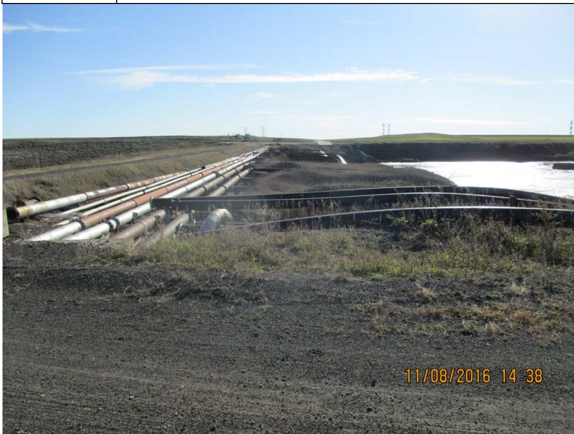
Photo 14 Interior of east embankment, looking south
