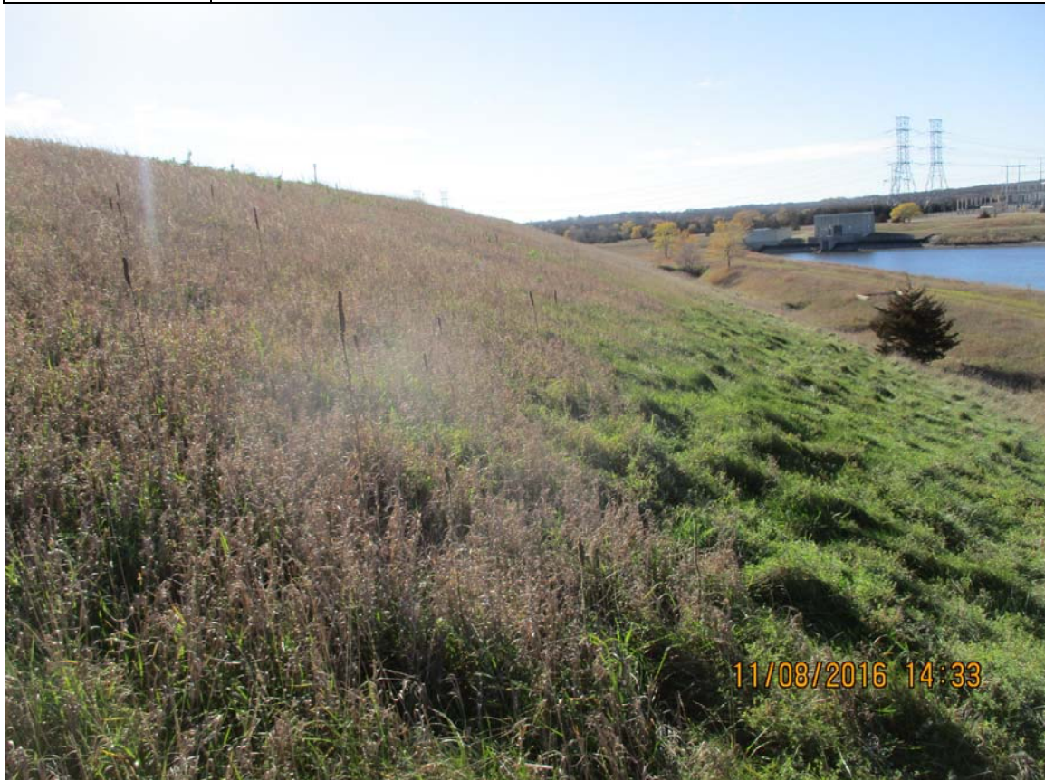
Photo 10 Mid slope of northwest embankment, looking southwest
