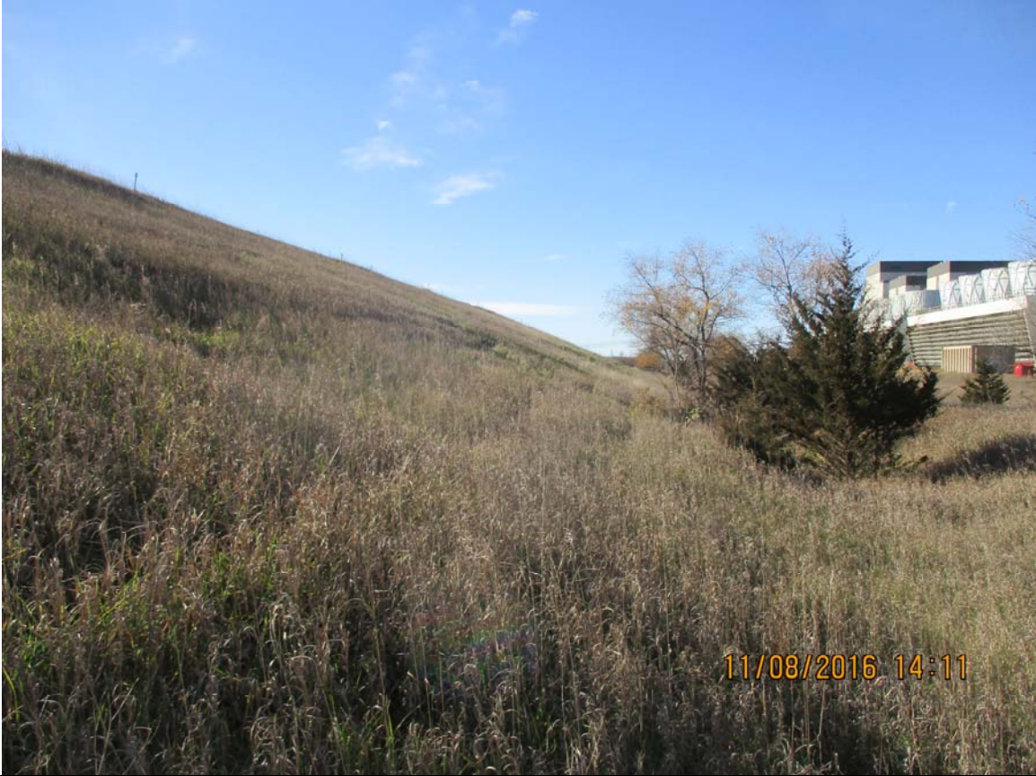
Photo 2 North embankment and perimeter ditch, looking west
