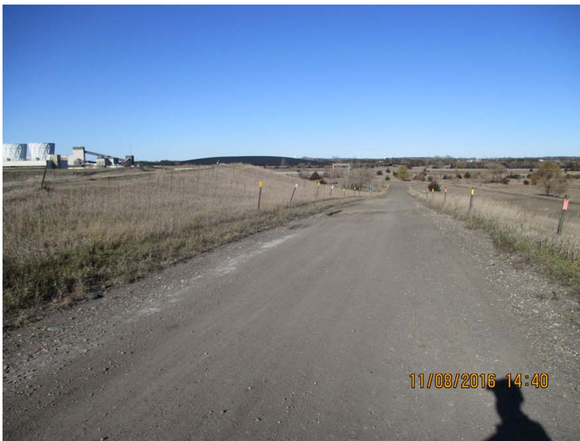
Photo 15 East embankment, looking north
