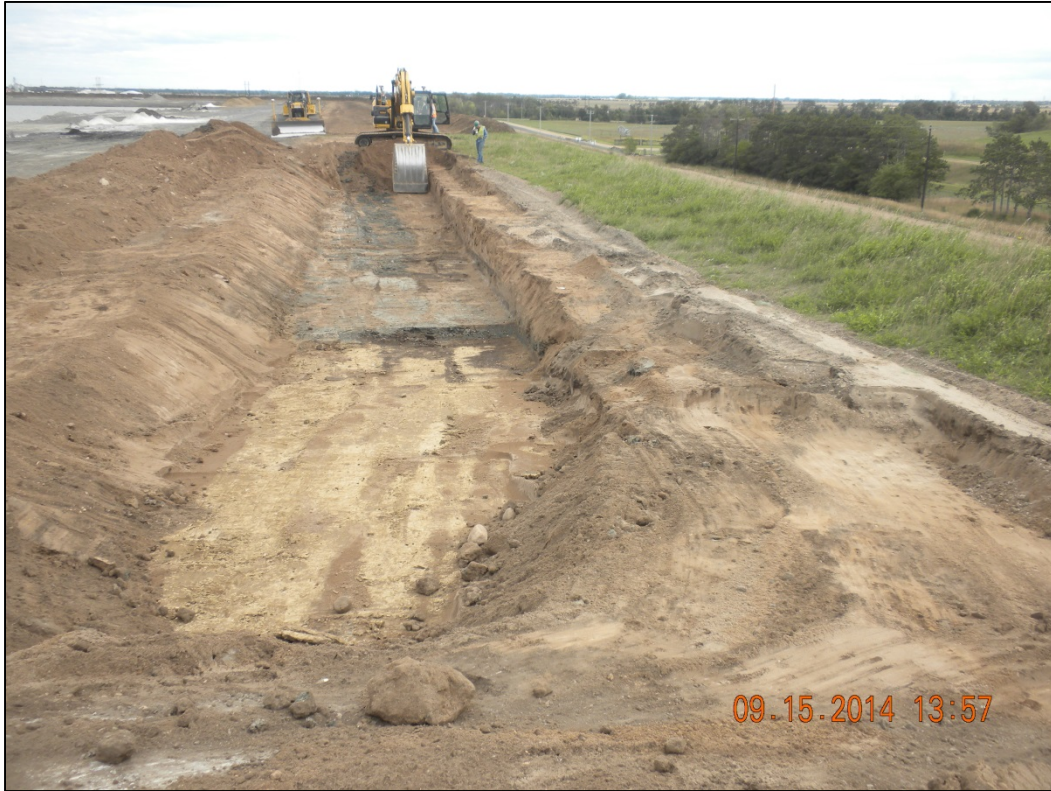
Photo 3: Exposing Existing Clay Barrier – Southwest Corner - Looking East – 9/15/14
