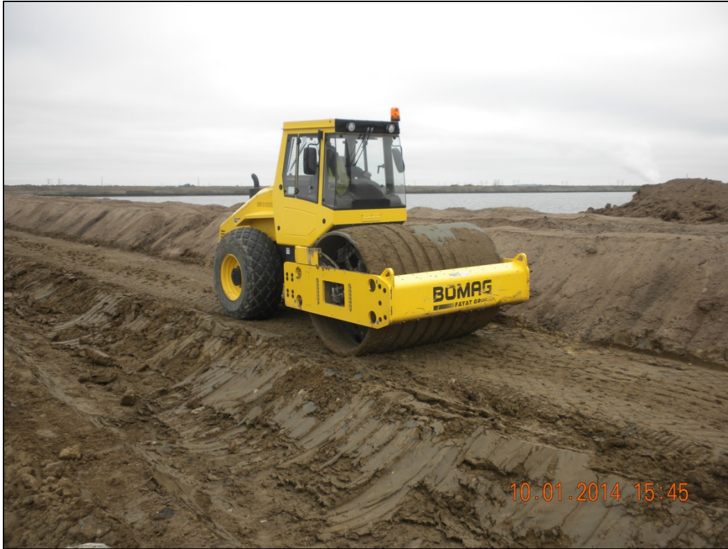
Photo 13: Smooth Rolling Top of Final Lift – East Section - 10/1/14
