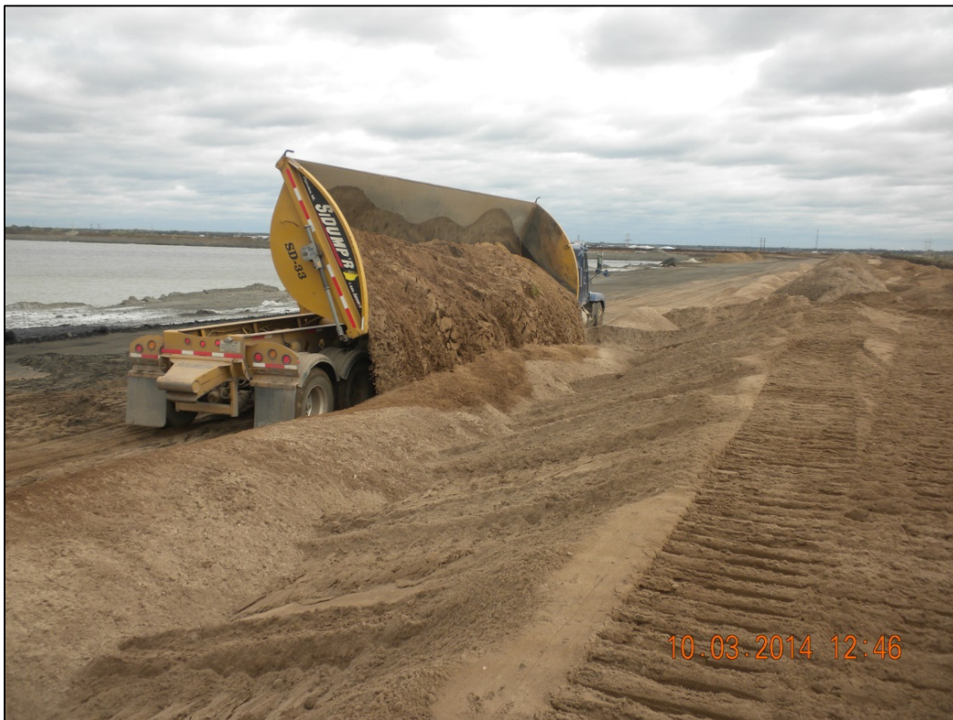
Photo 14: Placing Controlled Fill – South Berm Section - 10/3/14
