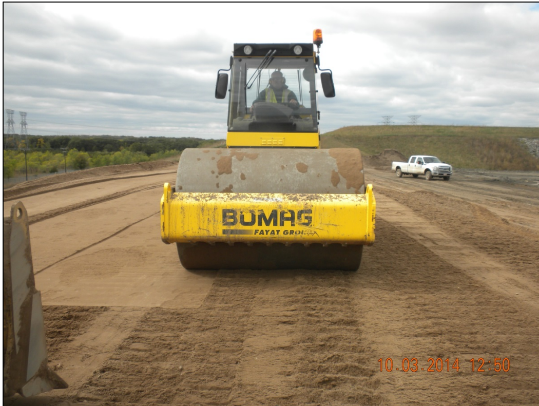
Photo 15: Compacting Controlled Fill – South Berm Section - 10/3/14
