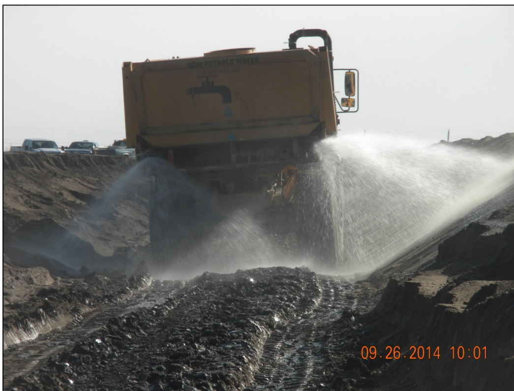
Photo 10: Watering Placed Clay - 9/26/14
