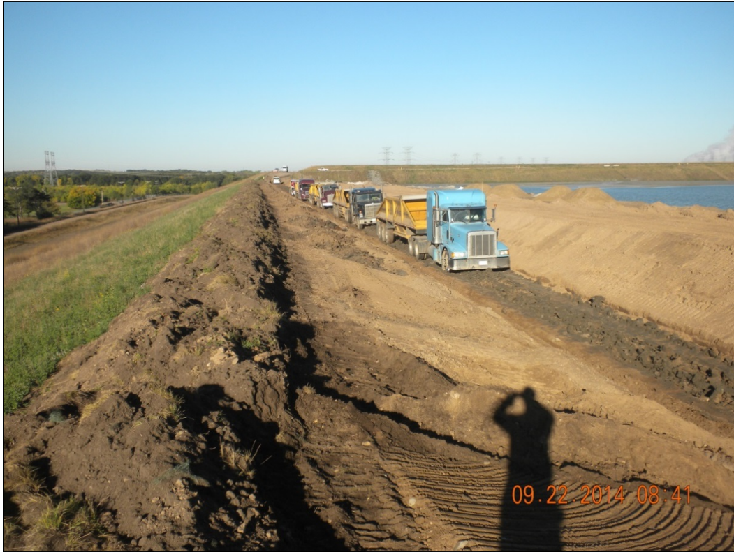
Photo 5: Placing Clay – South Berm Section – Looking West - 9/22/14
