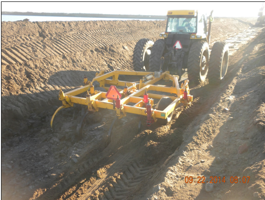
Photo 4: Scarifying Clay – South Berm Section - Looking East – 9/22/14
