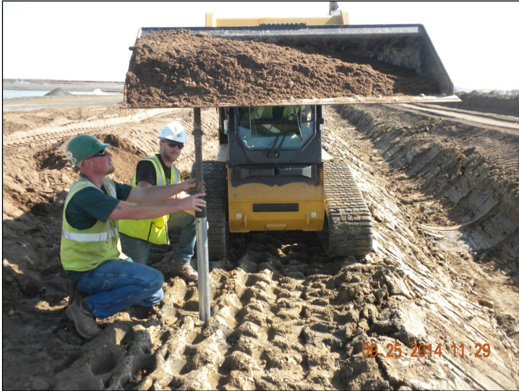
Photo 11: Clay Thin-Wall Sample Collection (CL TW-1) – Looking East - 9/25/14
