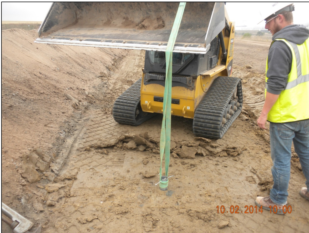
Photo 12: Clay Thin-Wall Sample Extraction (CL TW-2) – Looking West - 10/2/14
