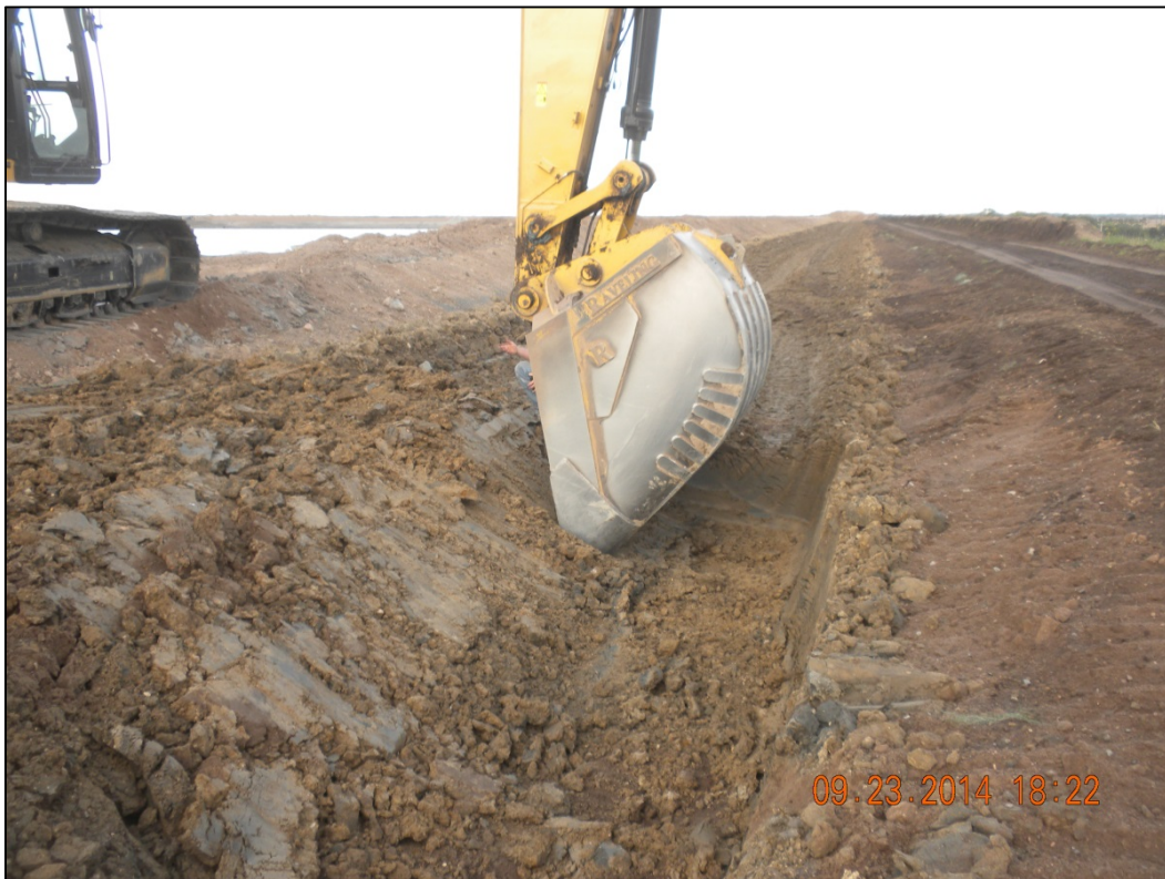
Photo 8: Lifting Outer Clay – Southeast Corner – Looking North – 9/23/14
