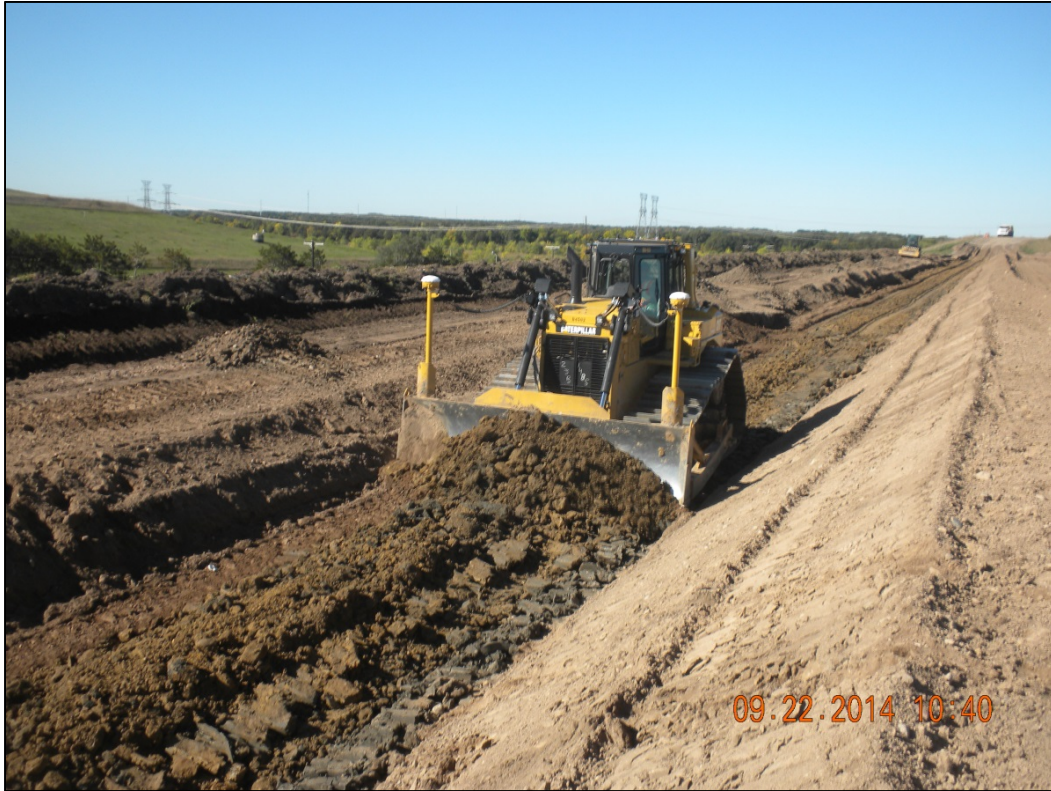
Photo 7: Grading Placed Clay – South Berm Section – Looking West - 9/22/14
