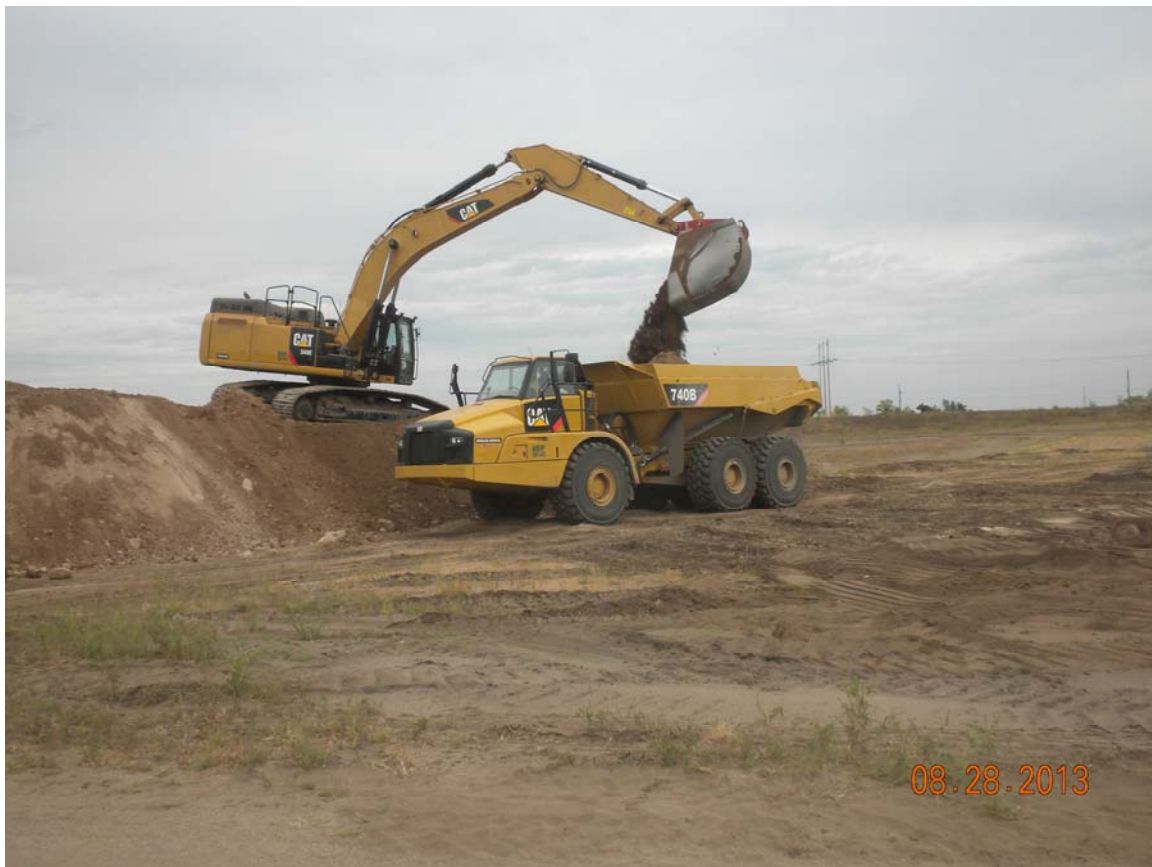
Photo 13 Backhoe loading off-road truck with random fill from the borrow area to be hauled to the Pond 3 South embankment. Looking northeast. 8/28/2013
