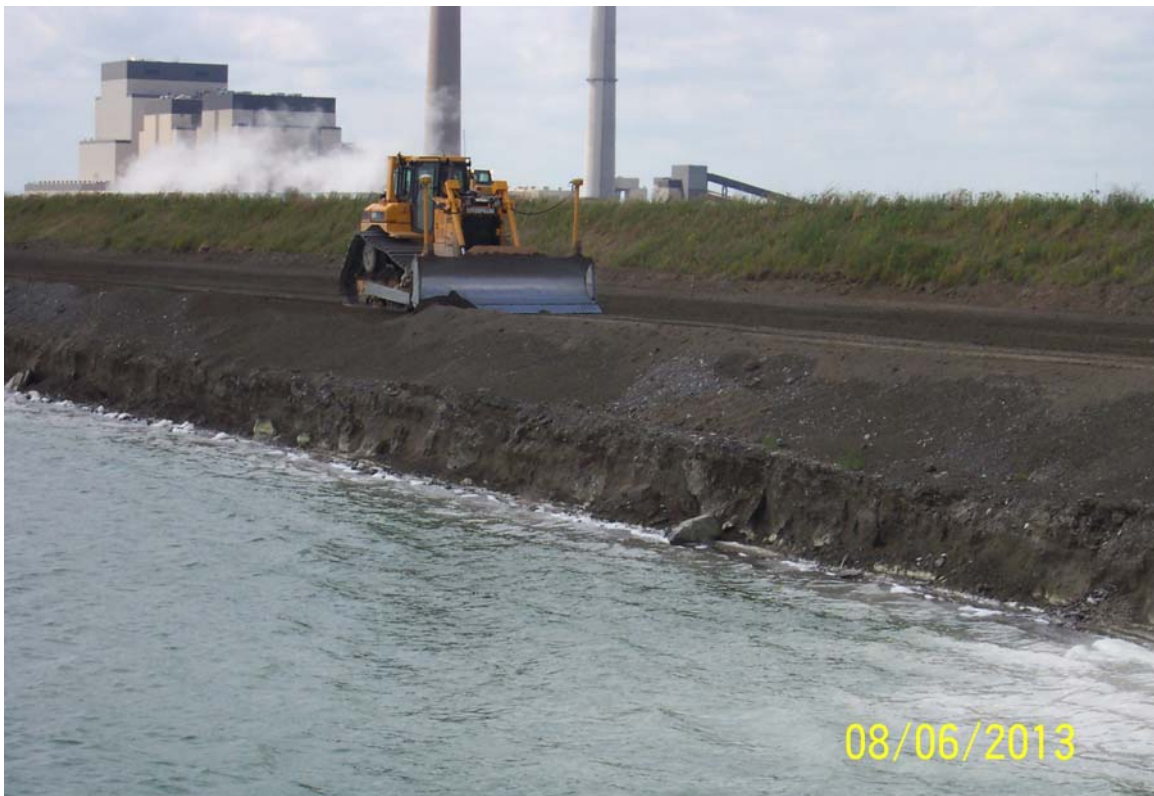
Photo 18 GPS dozer grading bottom ash on Pond 3 North in lifts. Looking northwest. 8/6/2013
