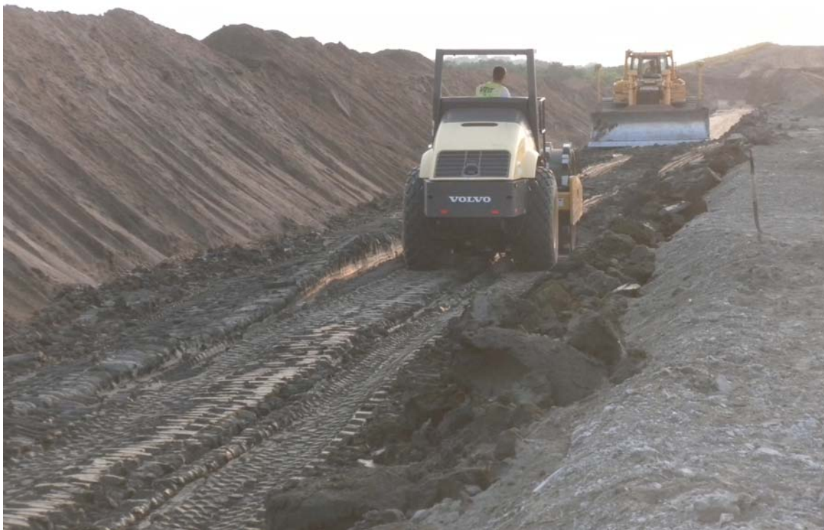
Photo 9 Right: Dozer spreading clay placed by belly dumps and side dumps into lifts. 8/19/2013 Middle: Vibratory sheepfoot roller compacting clay lifts. Looking west.
