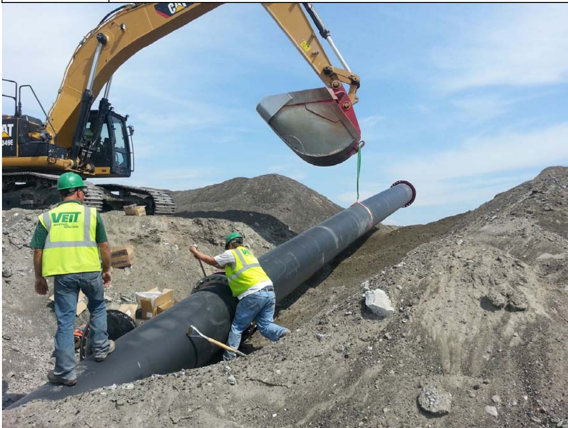
Photo 12 Foreground: Laborers bolting extension of Pond 3S dewatering riser pipe. Background, backhoe raising pipe to grade. Looking northeast. 8/26/2013
