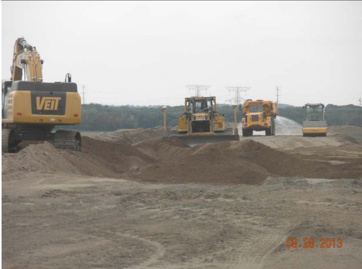
Photo 14 Left: Backhoe pulling random fill from exterior sideslope and placing on clay barrier. Middle Left: Dozer grading random fill in lifts over clay barrier. Middle Right: Water truck placing water on random fill. Right: Smooth drum roller compacting random fill. 8/28/2013
