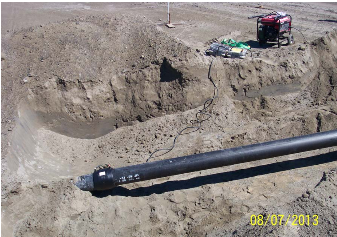
Photo 11 Electrofusion coupler used to extend 8-inch high density polyethylene cleanout pipe on the east side of Pond 3 South. Looking north. 8/7/2013
