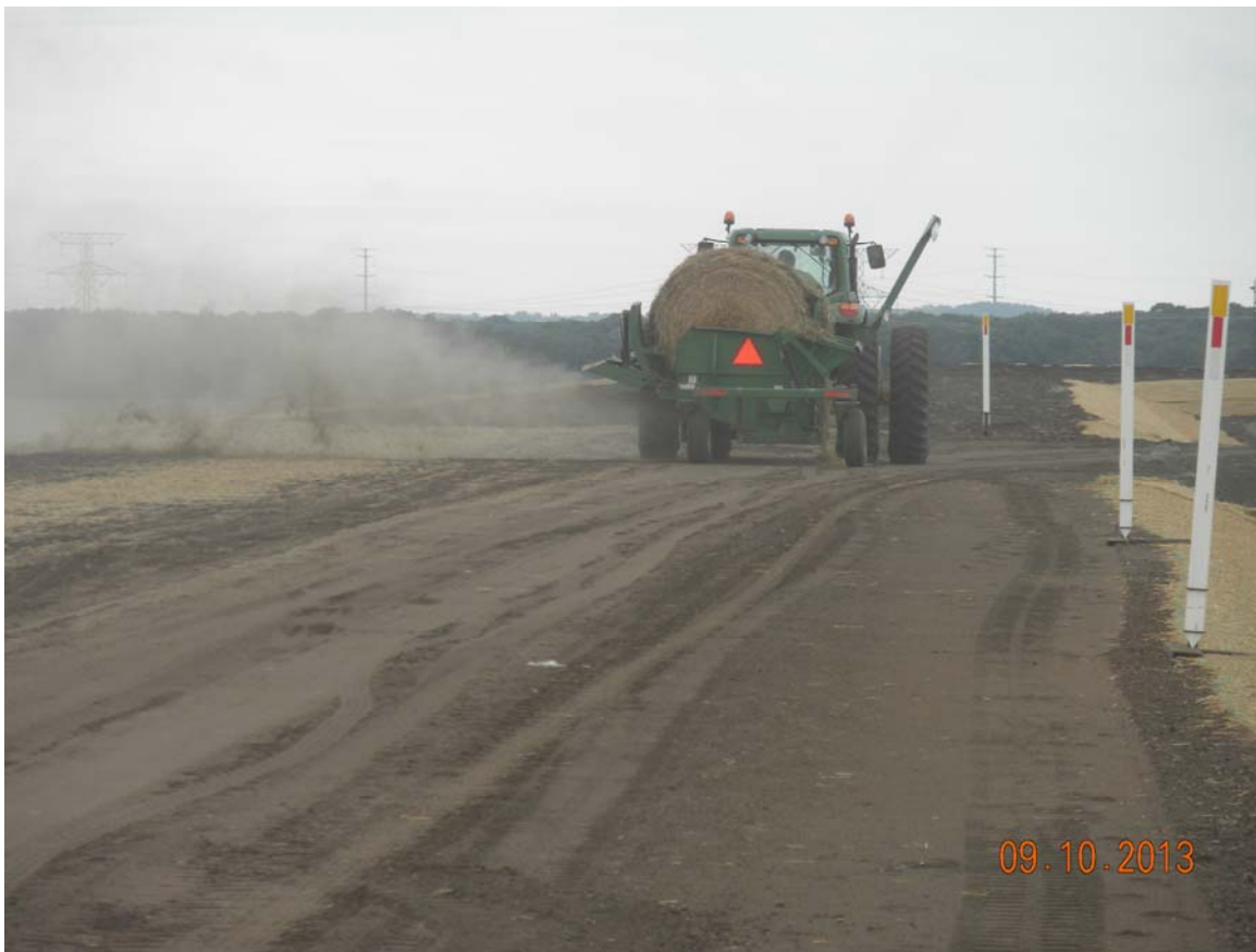
Photo 17 Tractor spreading mulch on top of top of the embankment. Looking south. 9/10/2013
