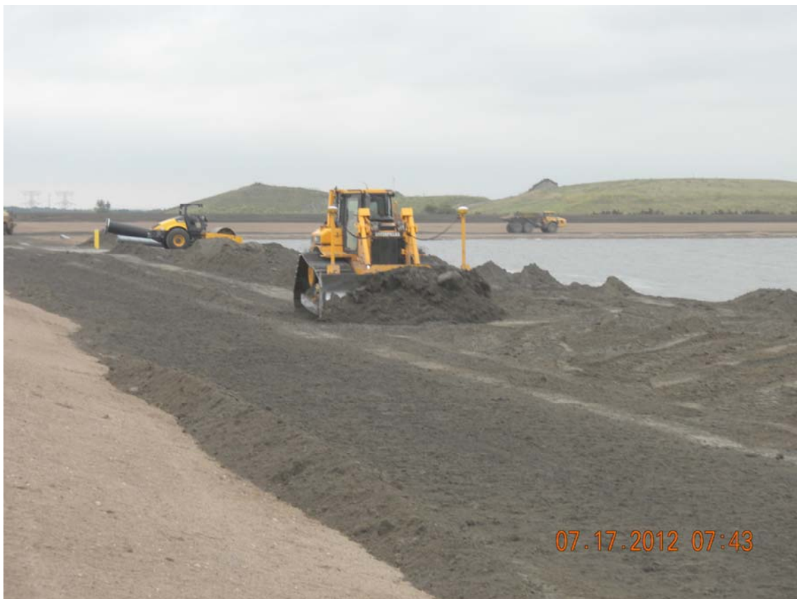
Photo 14 Dozer spreading bottom ash into lifts on the interior bench of Pond 3 South, looking south. 7/17/12
