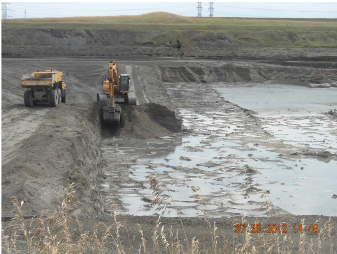
Photo 13 Backhoe excavating bottom ash to be hauled from the Bottom Ash Pond to Pond 3 South, looking south. 7/25/12
