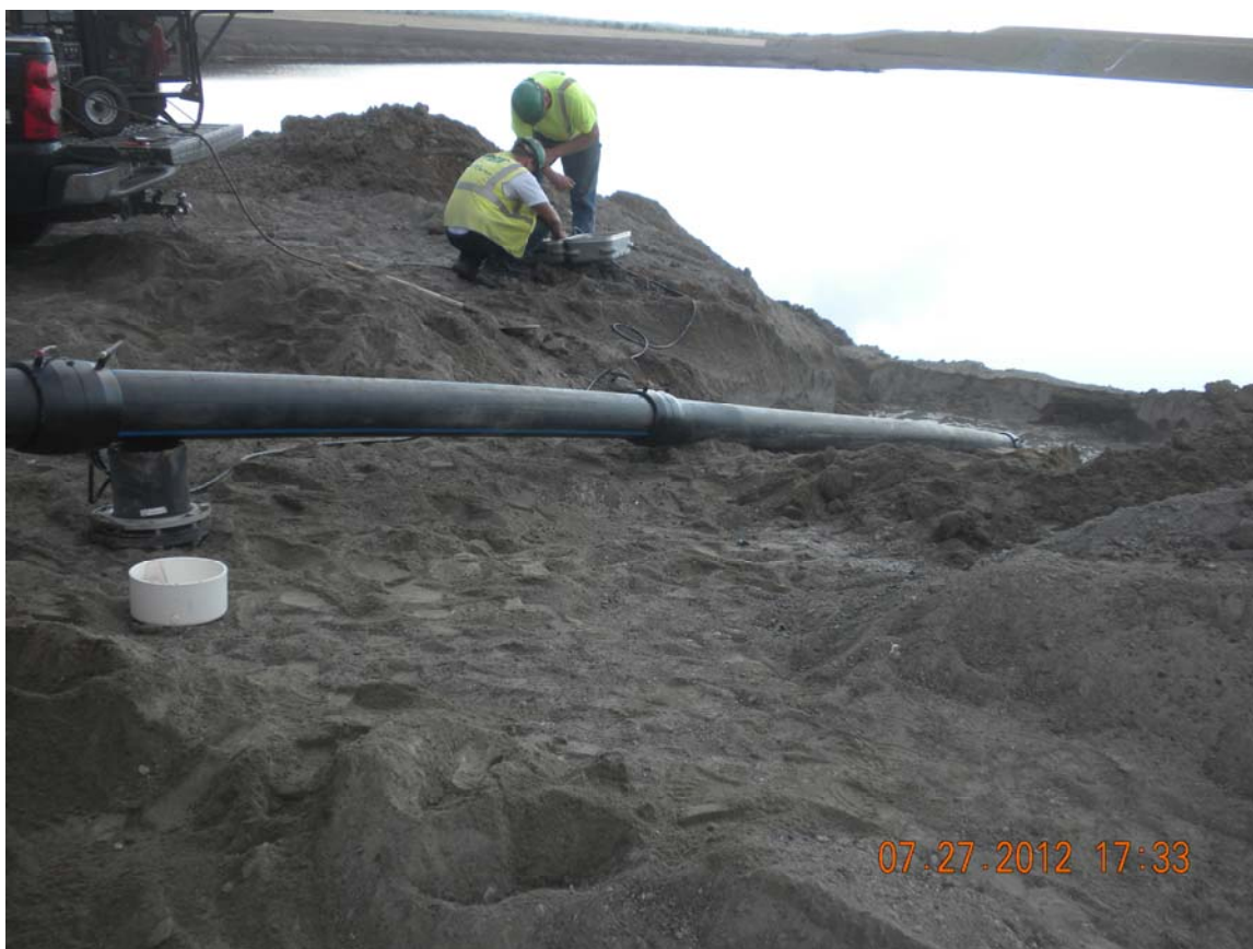
Photo 16 Laborers using electrofusion coupler to extend existing 8-inch high density polyethylene cleanout pipe on the east side of Pond 3 South, looking southwest. 7/27/12
