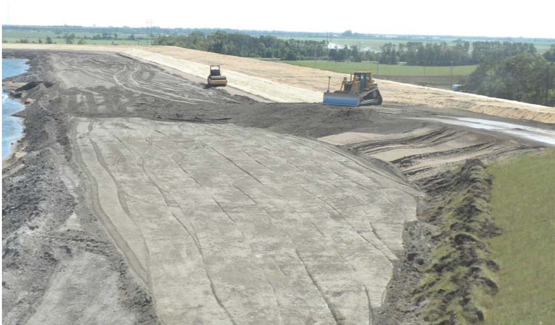
Photo 15 Compacted bottom ash on the south end of the interior bench, looking east. 7/26/12
