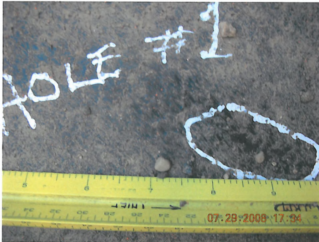
Photo 13: Hole #1 thin spot in membrane ~ 1- inch
