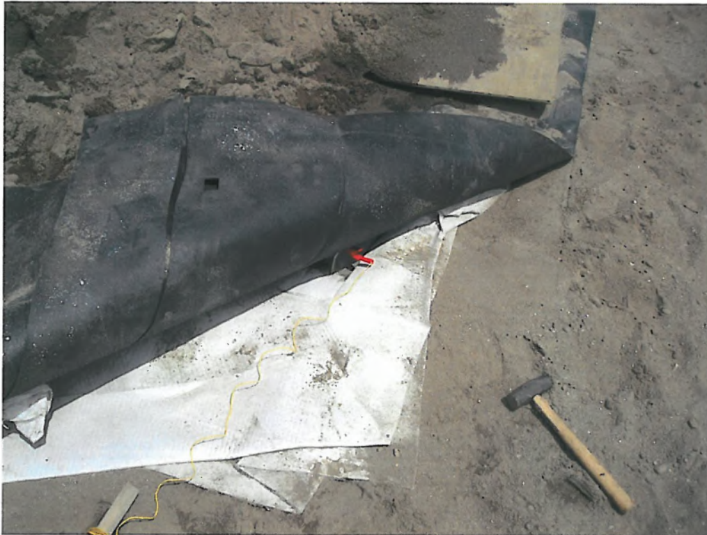
Figure 15: Ground pounded into GCL under membrane
