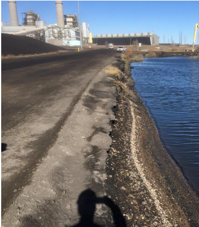
Comanche Station, Pueblo County, Colorado
