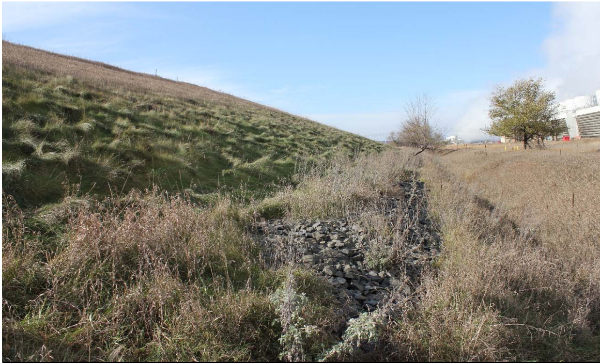
Photo 3 North embankment and riprap toe drain, looking west. 11/8/2017
