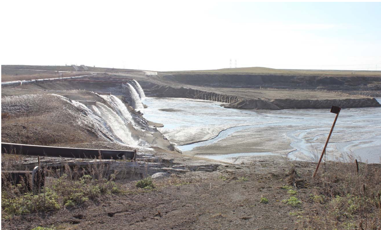
Photo 12 Pond interior, looking southeast. 11/8/2017
