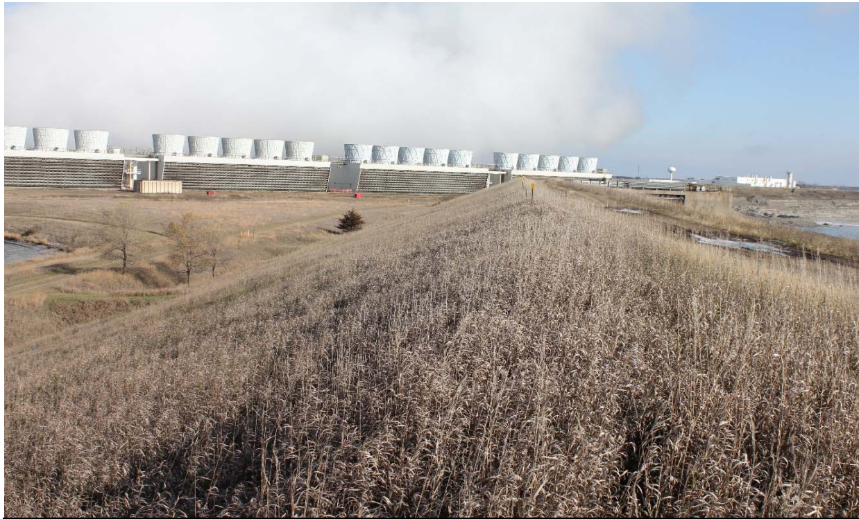
Photo 7 Northwest embankment, looking northeast. 11/8/2017
