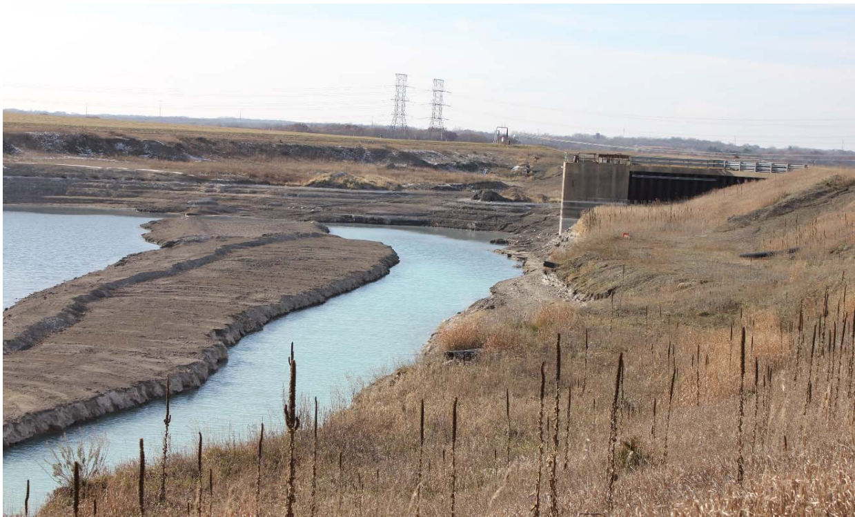
Photo 11 Pond interior, looking southwest. 11/8/2017
