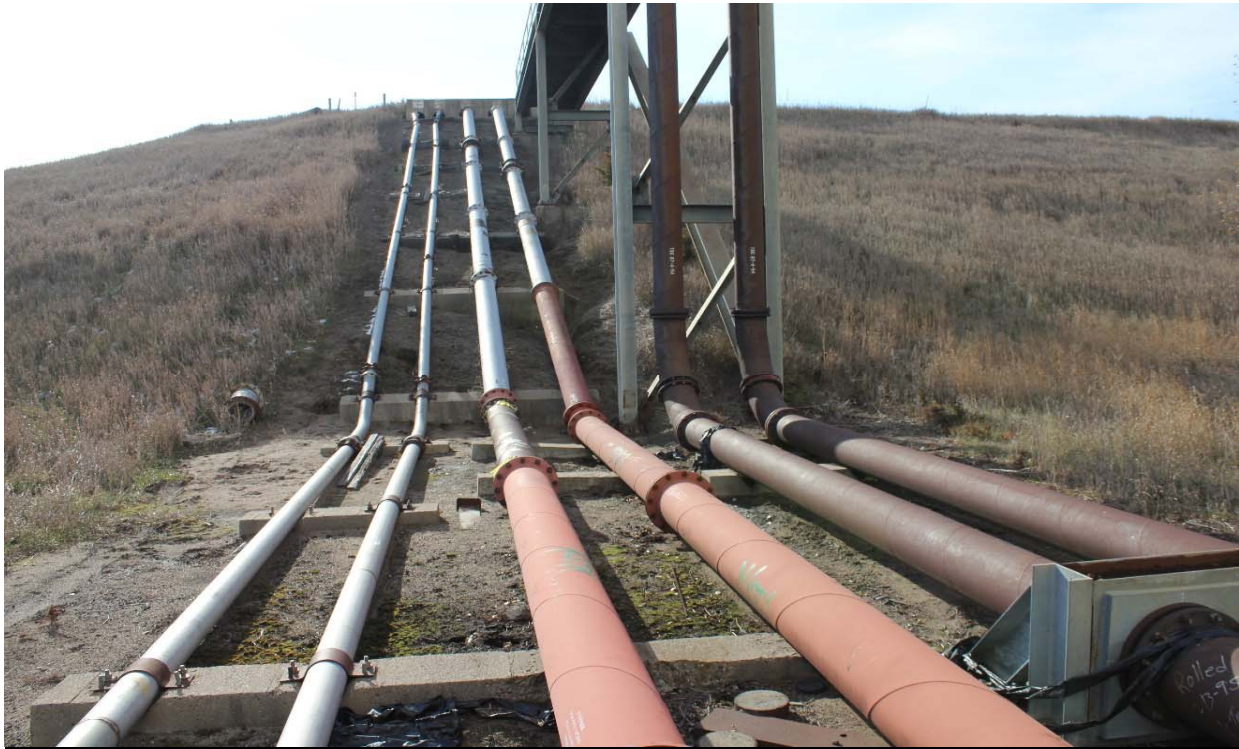
Photo 1 Bottom ash and scrubber pipes, looking south. 11/8/2017
