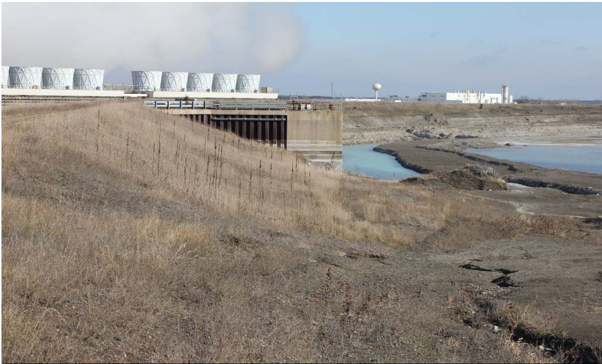
Photo 8 Pond interior, looking northeast. 11/8/2017
