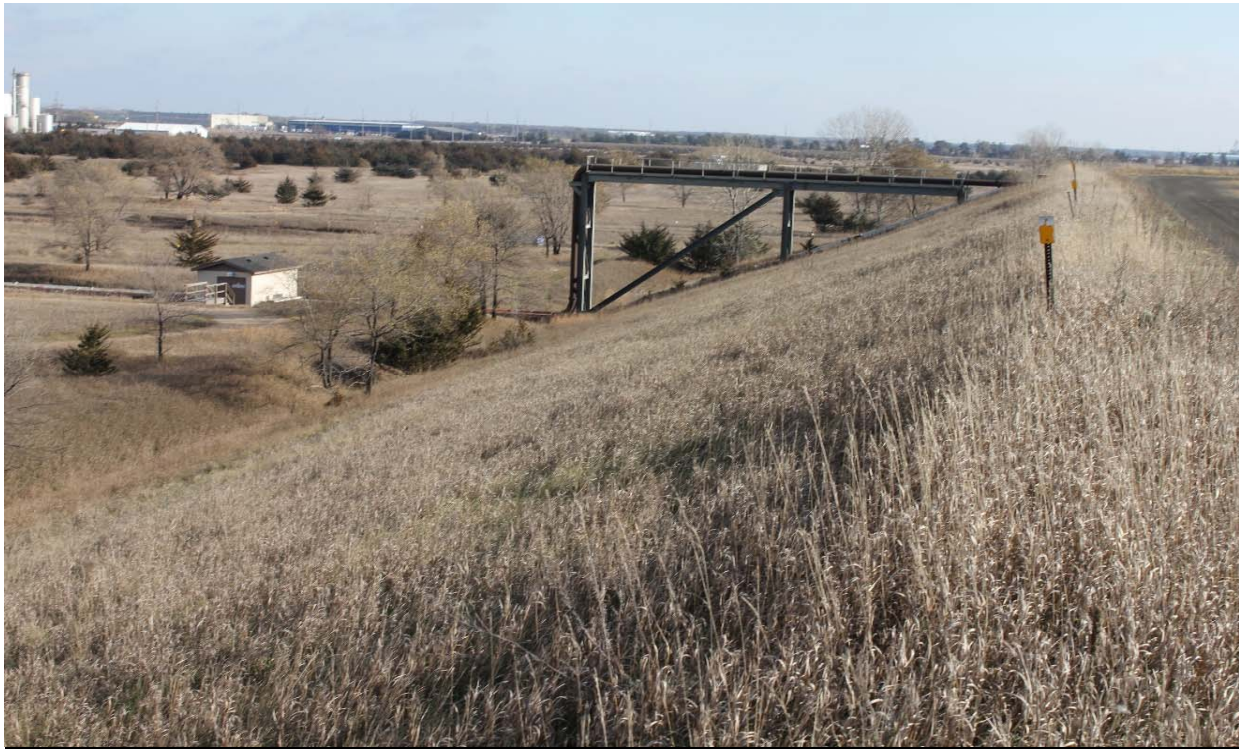
Photo 13 Upper slope of north embankment, looking east. 11/8/2017
