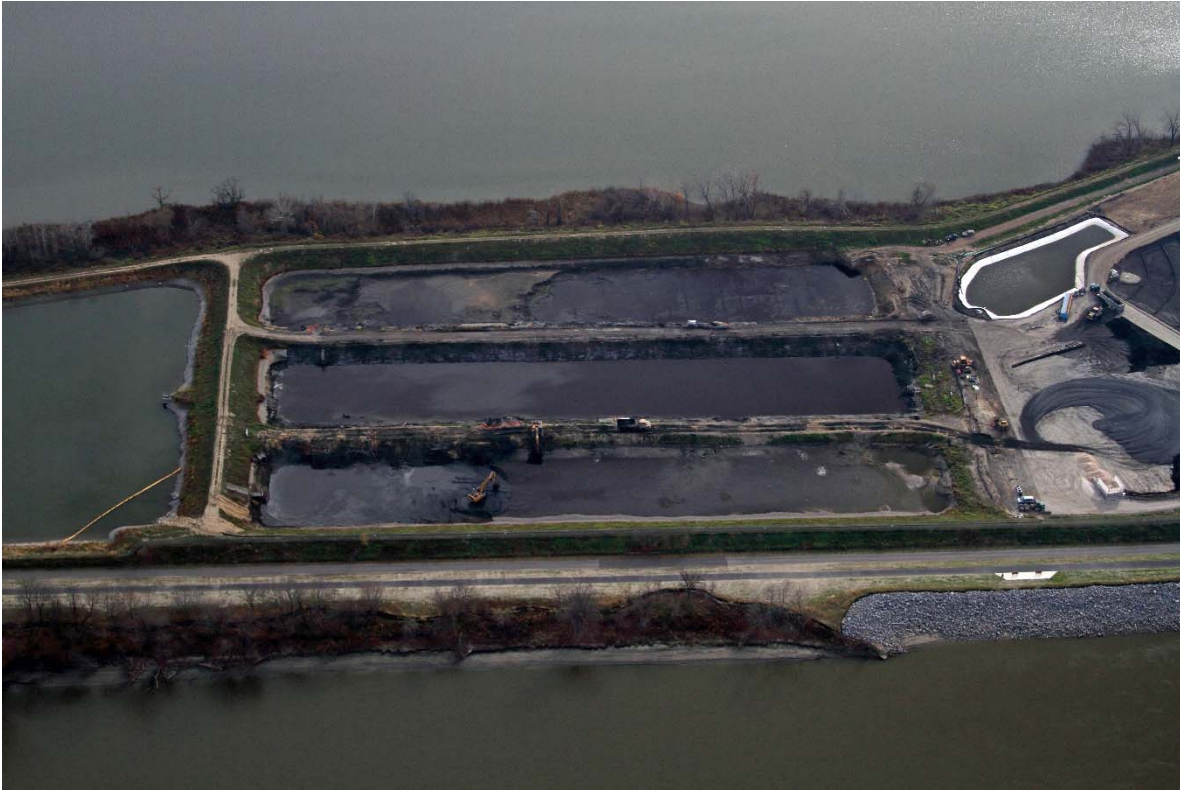
11/15/16 - Photo A-3: (Dredging in process)
