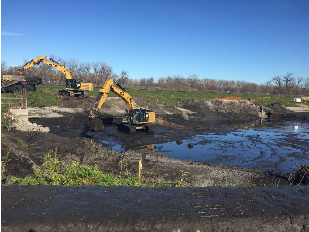
11/01/16 - Photo 2-5: (looking northeast)
