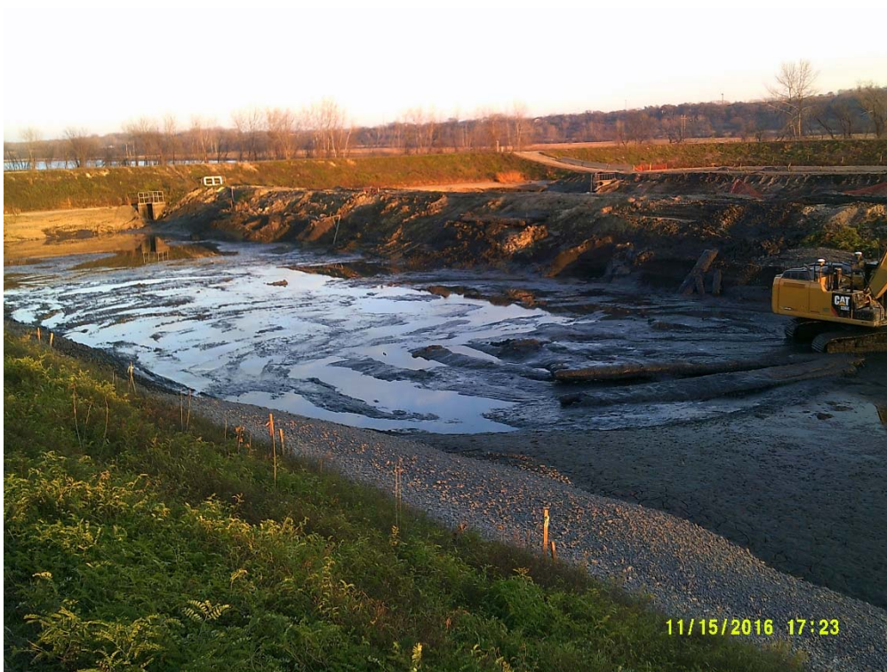
11/15/16 - Photo 1-5: (looking southeast)
