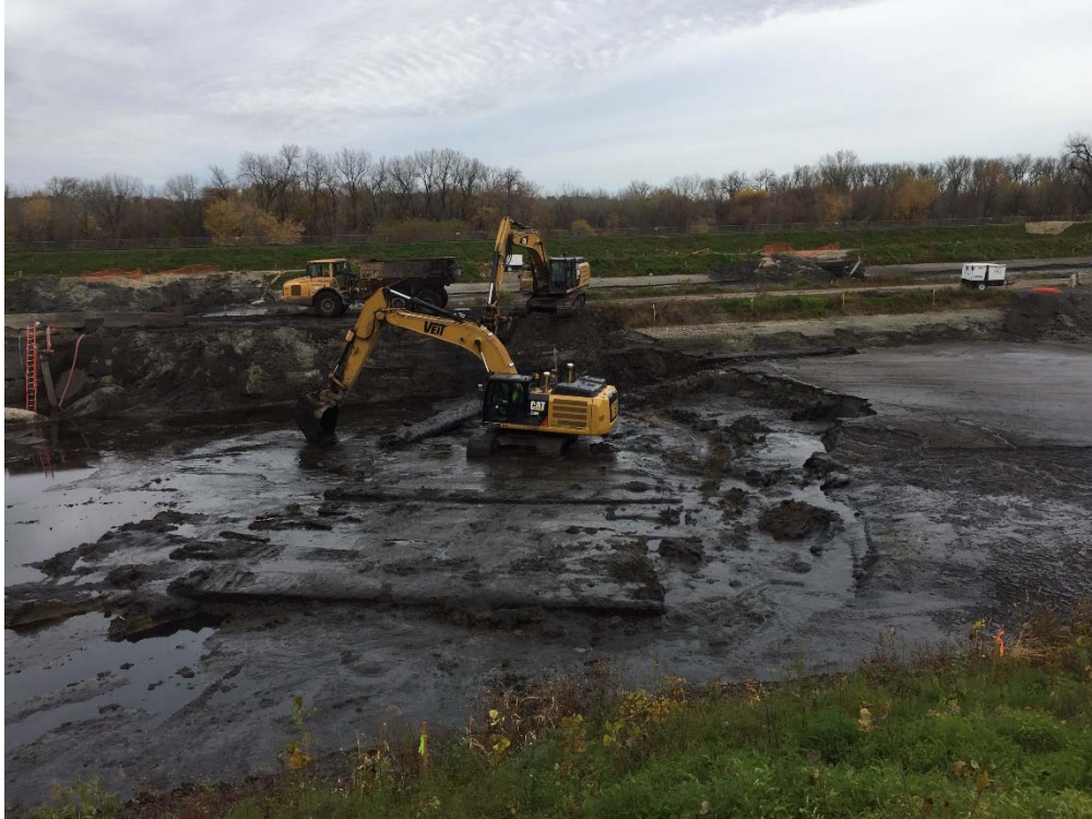
10/25/16 - Photo 3-9: (looking northeast)
