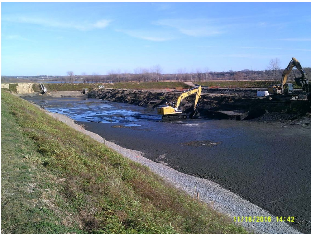
11/16/16 - Photo 1-6: (looking southeast)
