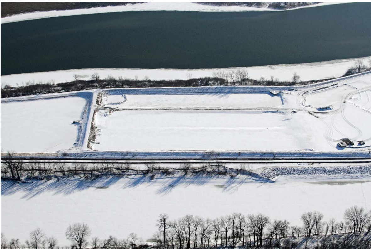
01/18/17 - Photo A-4: (Dredging completed)
