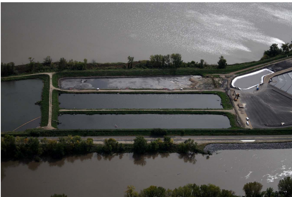
09/27/16 - Photo A-2: (Pond 3 dewatered prior to start of dredging)
