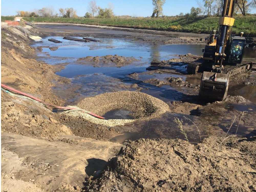
10/13/16 - Photo 3-5: (looking southeast)
