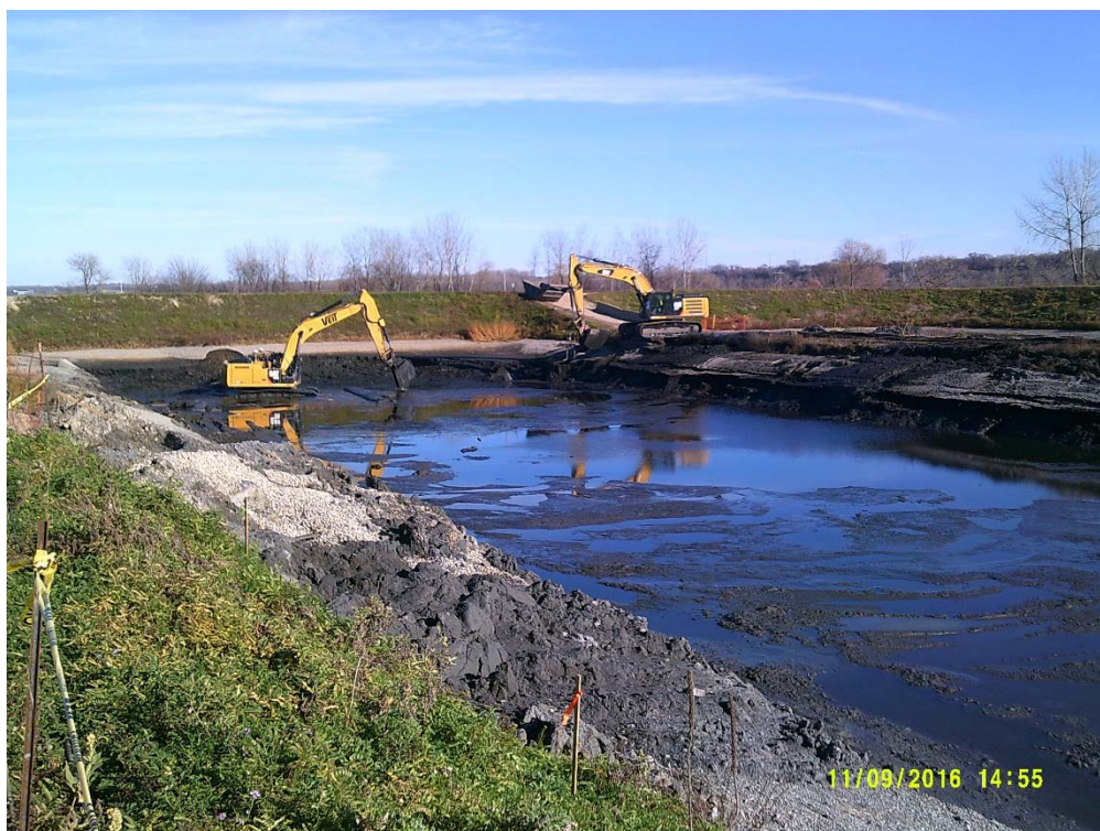
11/09/16 - Photo 2-8: (looking southeast)
