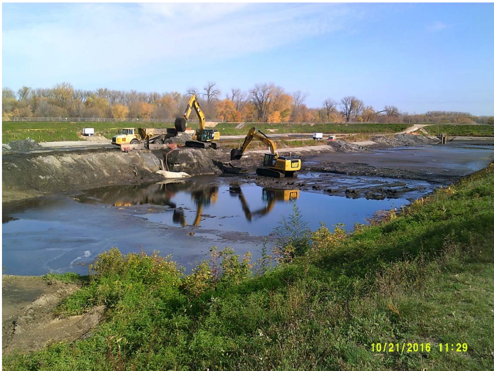
10/20/16 - Photo 3-8: (looking northeast)
