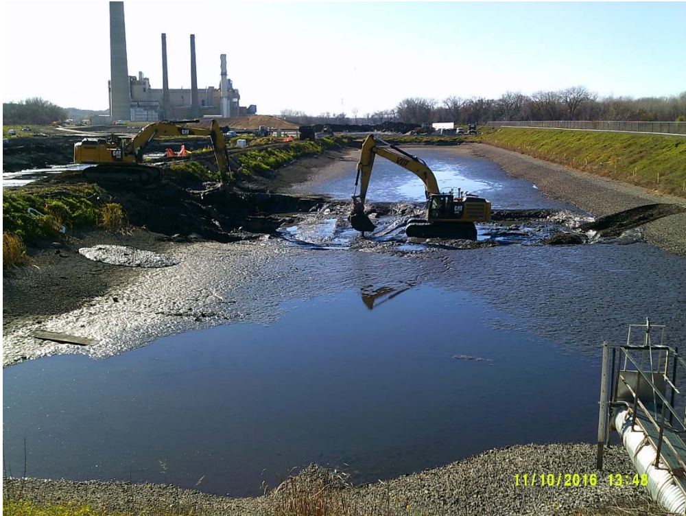
11/10/16 - Photo 1-3: (looking west)
