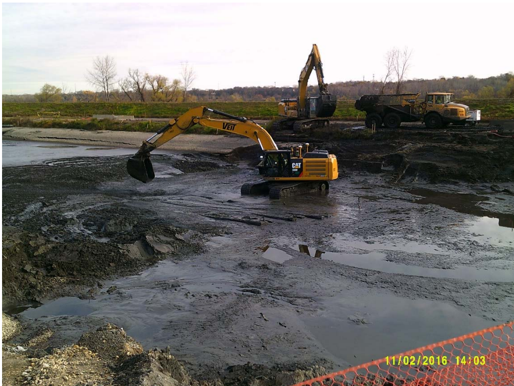
11/02/16 - Photo 2-6: (looking southeast)
