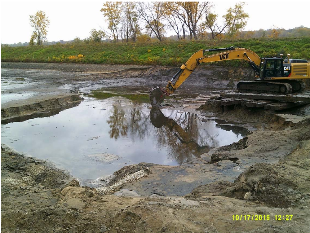
10/17/16 - Photo 3-6: (looking southeast)
