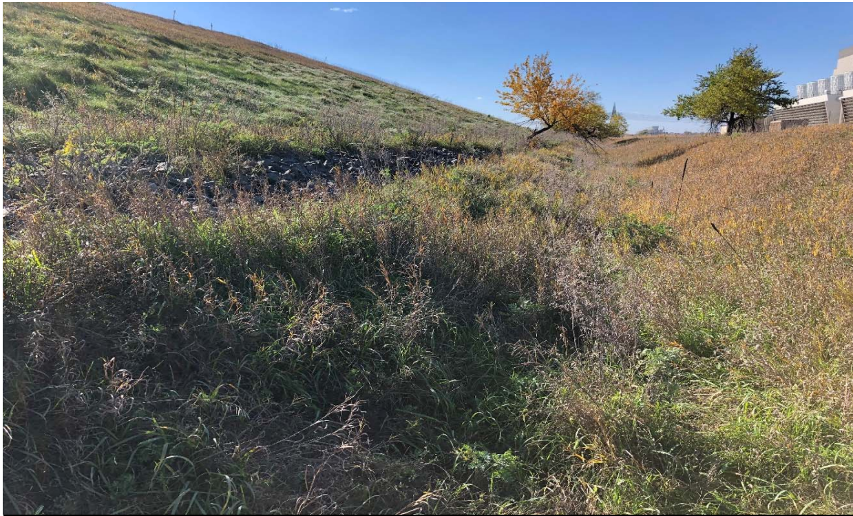
Photo 3 North embankment and riprap toe drain, looking west. 10/22/2018
