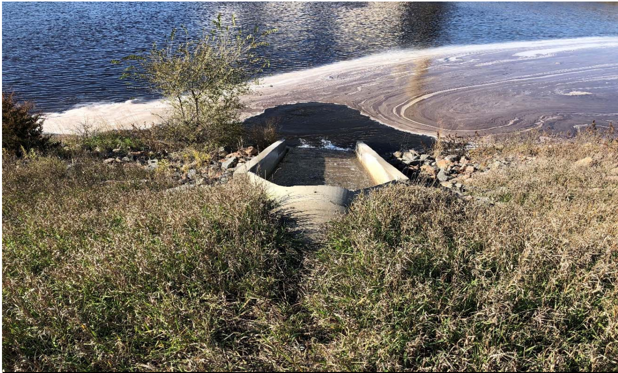
Photo 5 Bottom Ash Pond secondary outlet to Recycle Basin (Primary outlet is below the water level of the Recycle Basin). 10/22/2018
