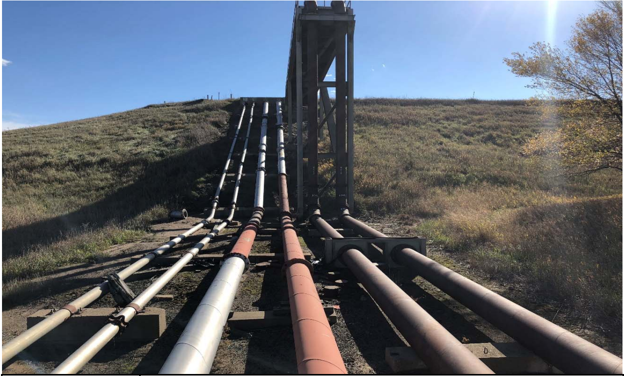
Photo 1 Bottom ash and scrubber pipes, looking south. 10/22/2018
