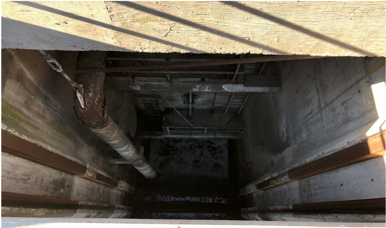
Photo 9 Photo from inside the discharge structure. Shows stop-log metal channels 10/22/2018 and water flowing over concrete stop-log at the bottom of the channel.
