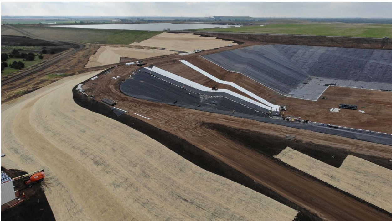
Photo 2 – Northeast corner of BAP2 during liner construction, looking southeast
