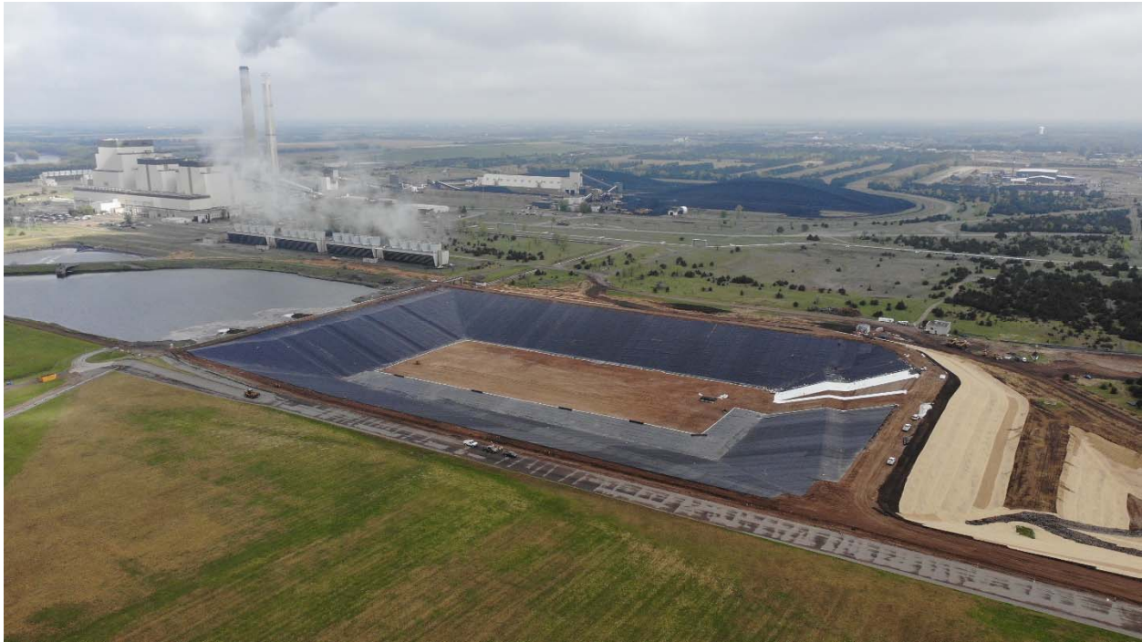
Photo 1 – BAP2 Liner Construction, looking Northwest (from Drone)
