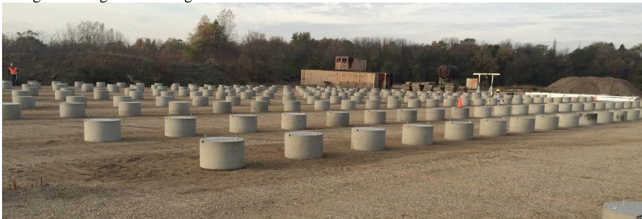
Pier placement prior to installation of racking
