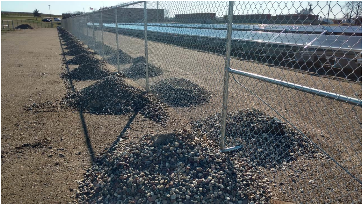
T-post fencing with ballast rock installed
