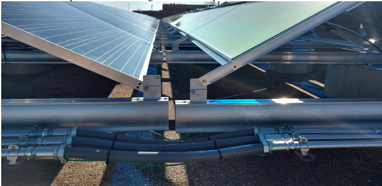
Rail mounted to pier with flexible conduit
