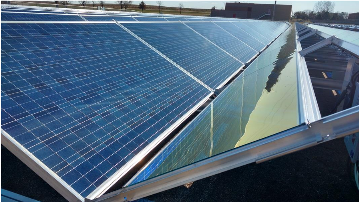
Reflective panels adjacent to solar PV panels
