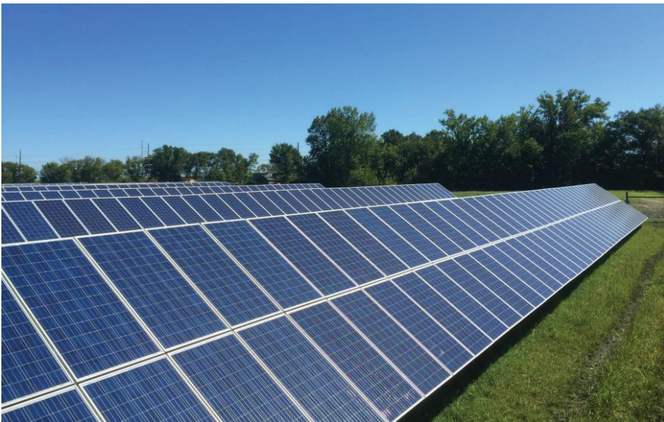
School Sisters of Notre Dame – 849 kW installation in Mankato was first large-scale array to use a 1,000 VDC platform in Minnesota.
