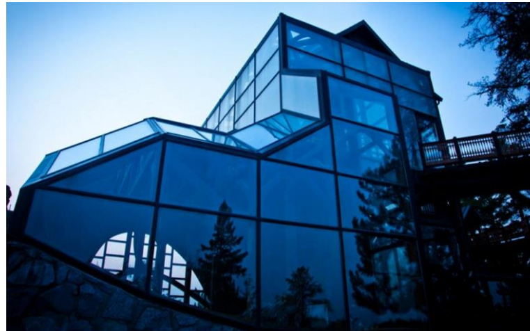
The Steger Wilderness Center is made of glass, native timber and stone, and recycled wood.
