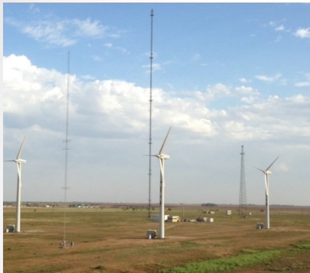
The DOE/SNL SWiFT Facility in Lubock, TX
