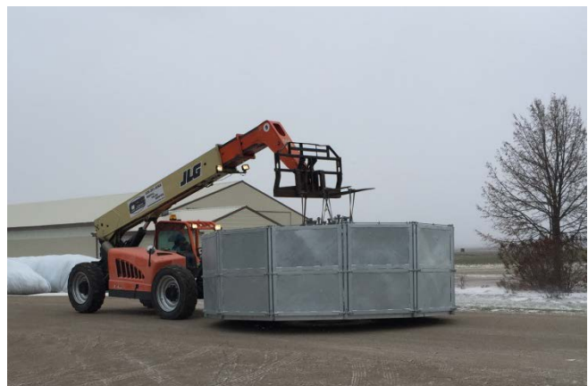
Figure 5. Bringing Tower Foundation to Site
