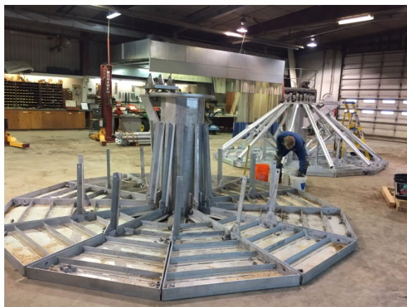
Figure 5. Wind Tower Foundation Assembly
