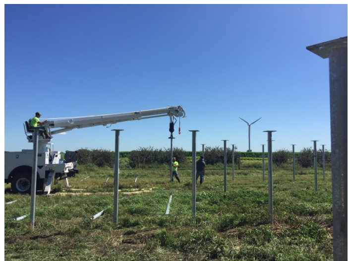
Figure 1. Installing Solar Array Earth Anchors
