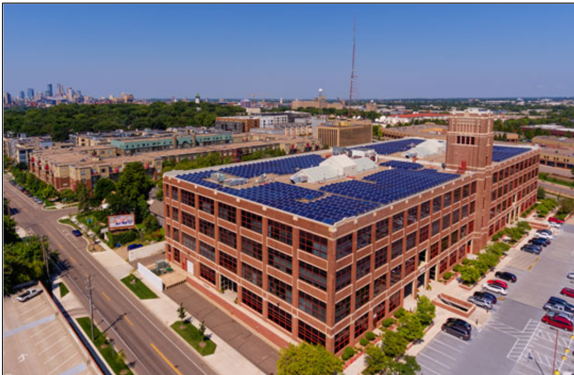
2550 University Avenue Completed Installation
