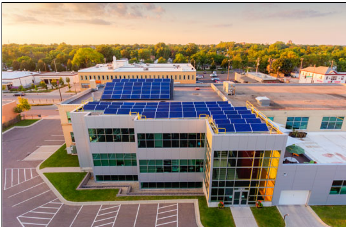
1000 University Avenue Completed Installation
