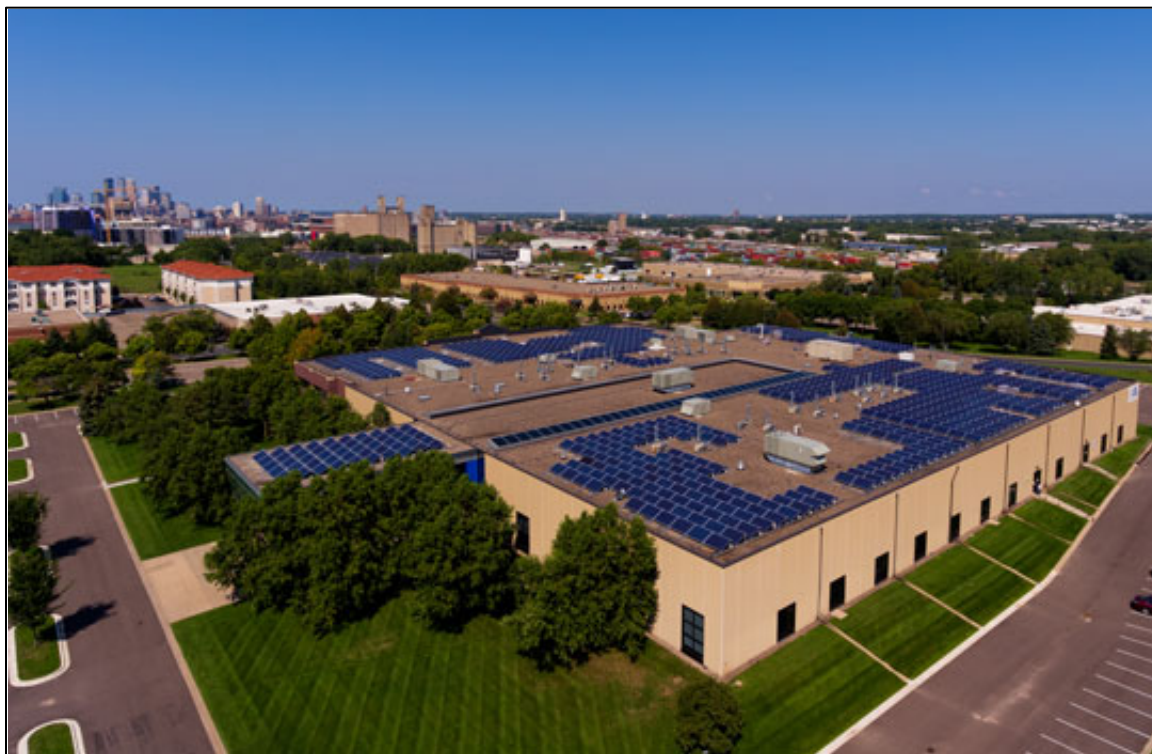
1000 Westgate Completed Installation
