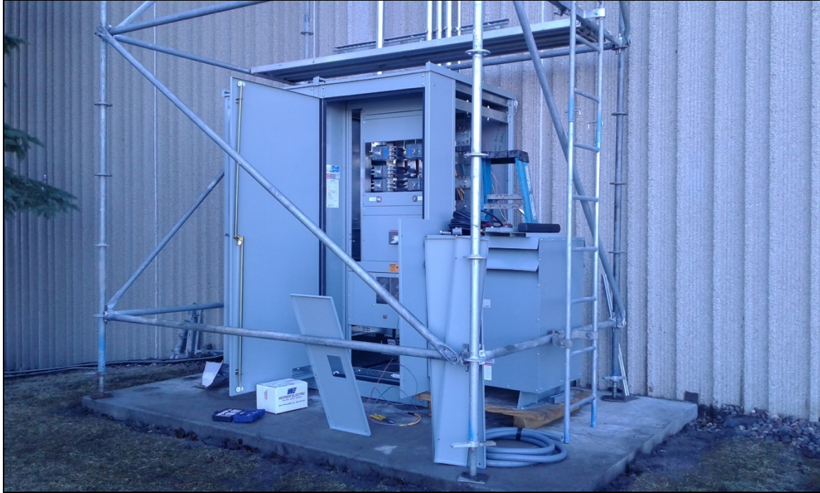
Switchgear Under Construction at 1000 Westgate Drive
