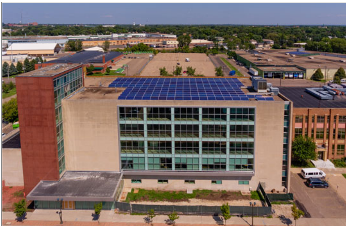
1919 University Avenue Completed Installation
