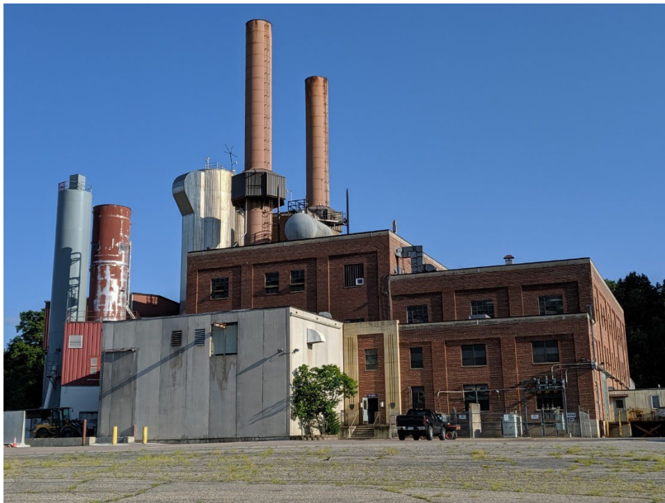
Figure W-2: Wilmarth Waste-to-Energy Generating Plant
