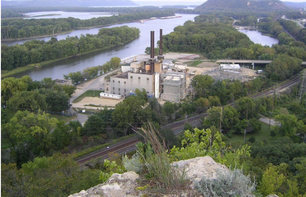
Figure W-1: Red Wing Waste-to-Energy Generating Plant
