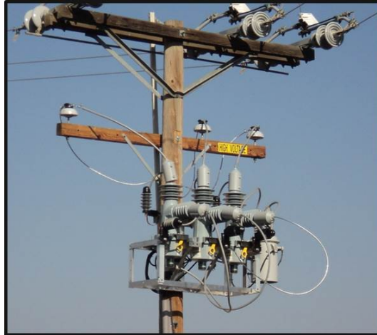
Figure CSN-D-12 Recloser on Distribution Pole
