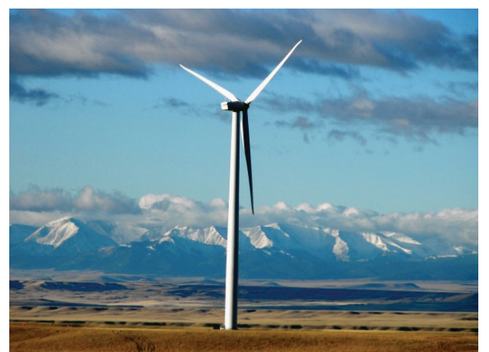
The Rush Creek project is expected to include 300 wind turbines. Each of the wind turbines will have an estimated capacity of 2 megawatts for a 600 megawatt total capacity. The turbine hub height is typically about 260 feet with the tip of the blade being approximately 440 feet tall.
