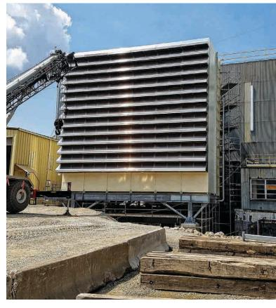
The most challenging part of the process involved configuring the new unit within the existing plant building at Black Dog, Danberg said. Modifications were needed in order to make the move-in possible.
