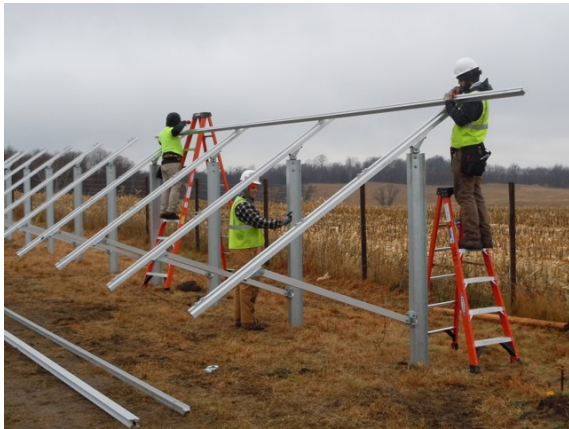
Racking Assembly
