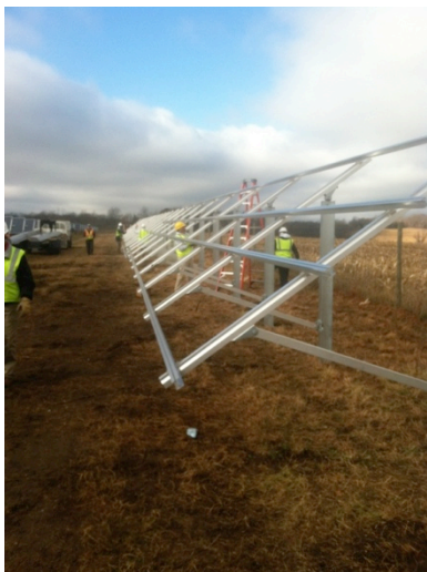
Racking Nearing Completion
