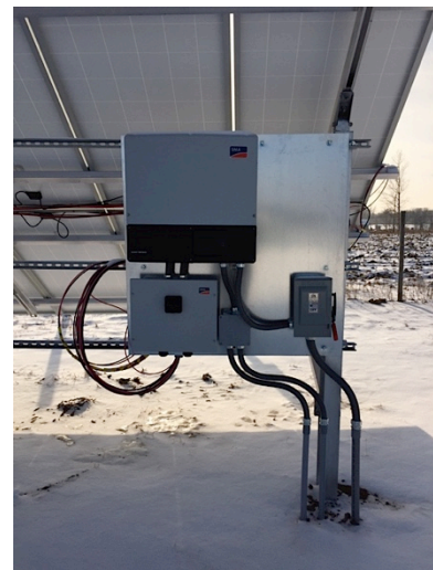
1 of 7 new 20kW Inverters
