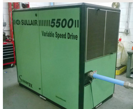
A new compressor featured high- and low-pressure options. Upgrades and efficiency measures resulted in savings of nearly 10 percent.
