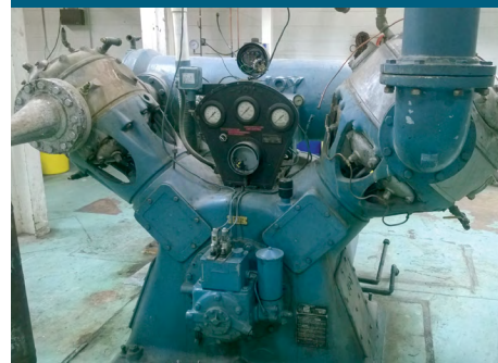
The piston compressor did not adapt to energy demand variables.
